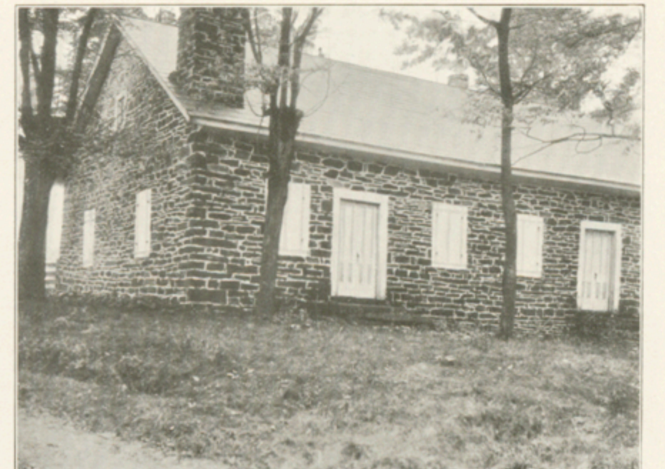
PLATE 20.—OLD QUAKER MEETINGHOUSE NEAR BERMUDEAN CHURCH Built in eighteenth century of Triassic red sandstone
