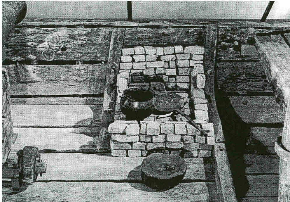
Figure 7-20. Recreation of the Hearth with Iron Cook Pot on Board 1776 American Vessel Philadelphia (Courtesy of the Smithsonian Institution from Bratten 1997:316)
