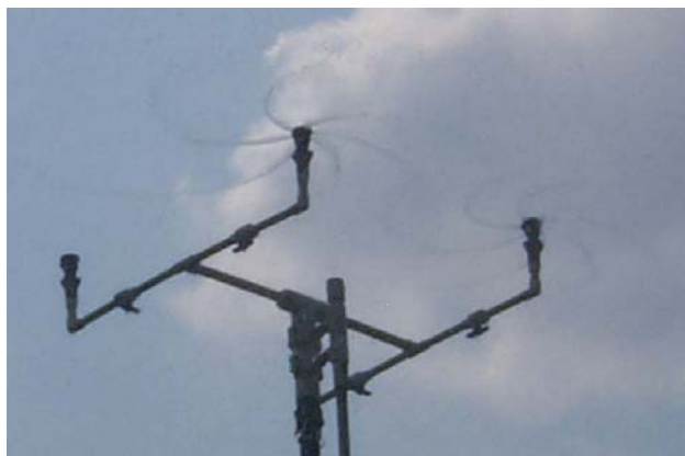
Figure 1. H-pattern sprinkler manifold operating during a test run.
