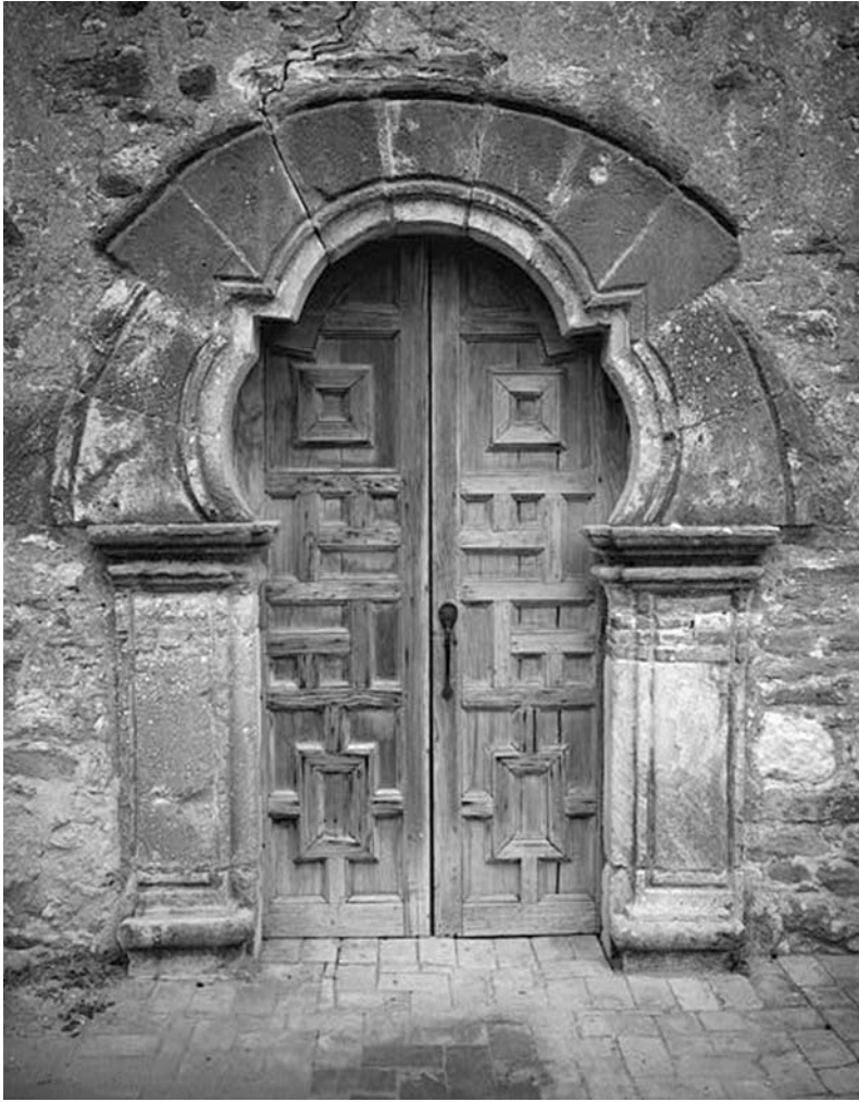
Fig. 14. Mission Espada church portal, showing herradura . (Library of Congress, Prints and Photographs Division, Historic American Buildings Survey, HABS TEX,15-SANT.V,2-A-6.)
