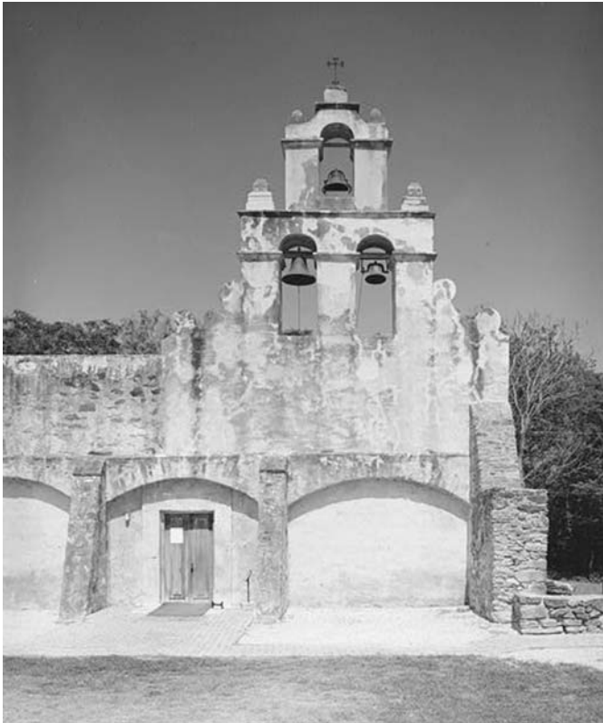
Fig. 13. Mission San Juan church façade, showing espadaña . (Library of Congress, Prints and Photographs Division, Historic American Buildings Survey, HABS TEX,15-SANT.V,3A-5.)
