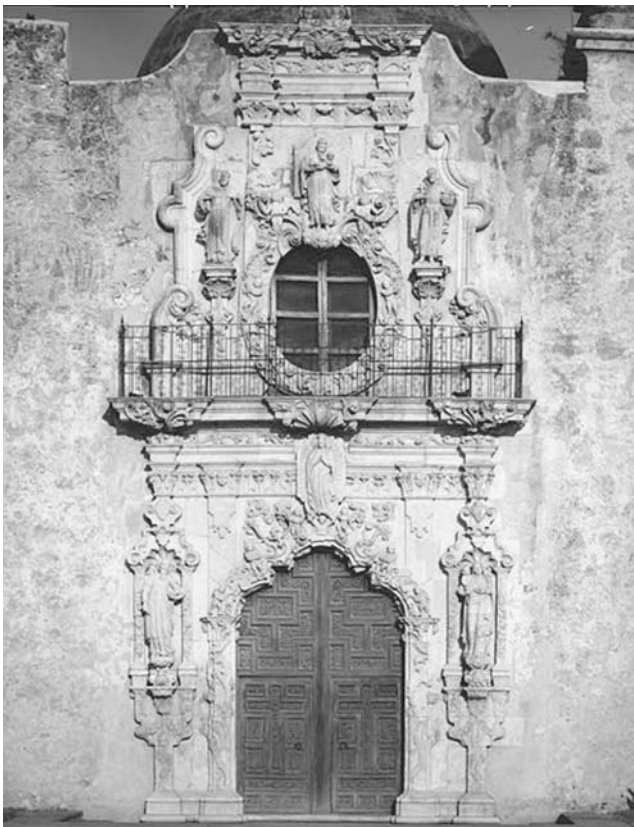
Fig. 9. Mission San Jose church portal. (Library of Congress, Prints and Photographs Division, Historic American Buildings Survey, HABS TEX,15-SANT,V,5E-6.)
