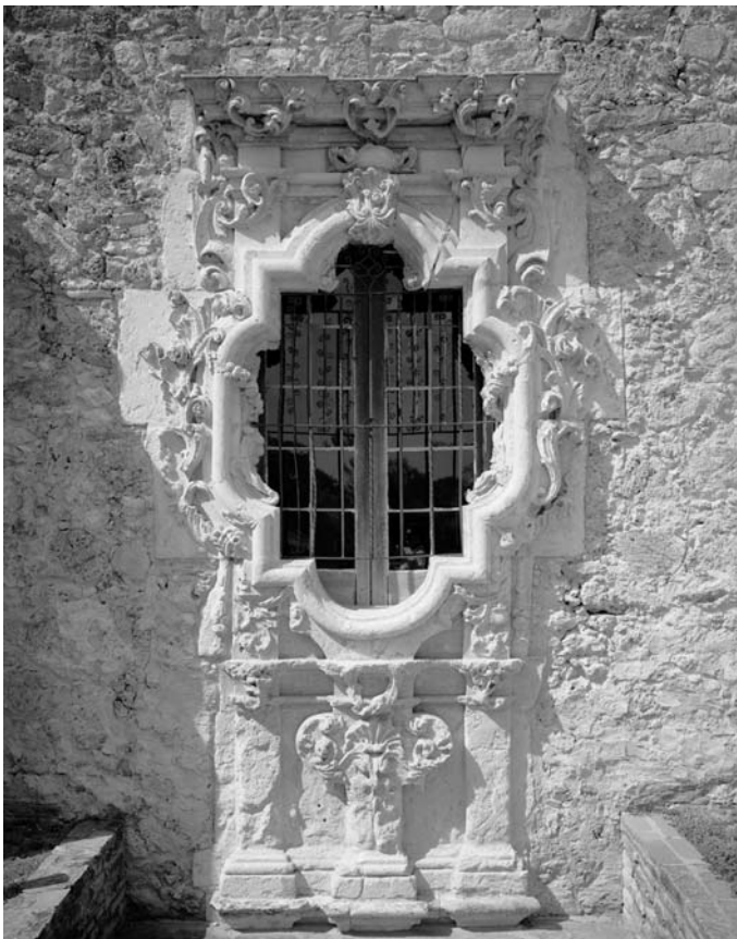
Fig. 10. Rose Window of the sacristy at Mission San Jose. (Library of Congress, Prints and Photographs Division, Historic American Buildings Survey, HABS TEX,15-SANT.V, 5F-2.)
