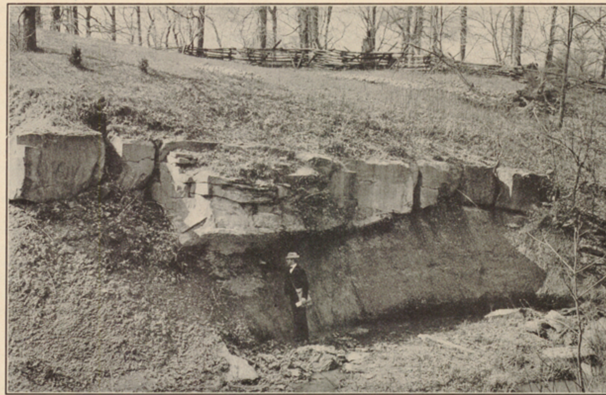
PLATE V.—BEREA SANDSTONE RESTING UNCONFORMABLY ON BEDFORD SHALE, NEAR LITHOPOLIS. The hard ledge above the man's head shows the full thickness of Berea sandstone present at this place. The nature of the unconformity and the variable thickness of the sandstone are clearly shown. (Photograph by H. A. Gleason.)
