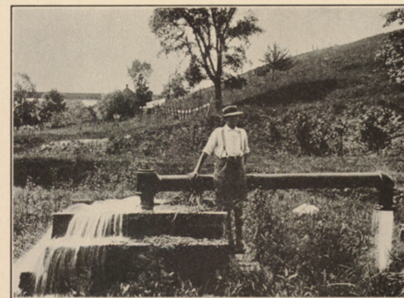
PLATE VIII.—FLOWING ARTESIAN WELL NEAR HARRISBURG. Water obtained from Silurian limestone about 400 feet below surface.
