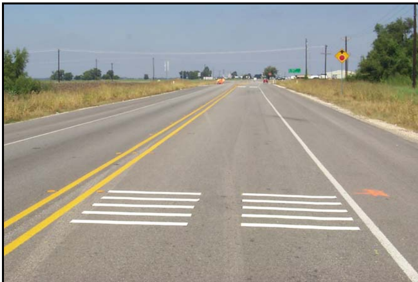
Figure 7. Upstream View of Installed Rumble Strips
