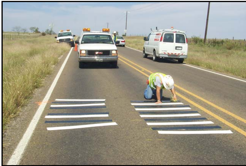
Figure 6. Installation of Rumble Strips
