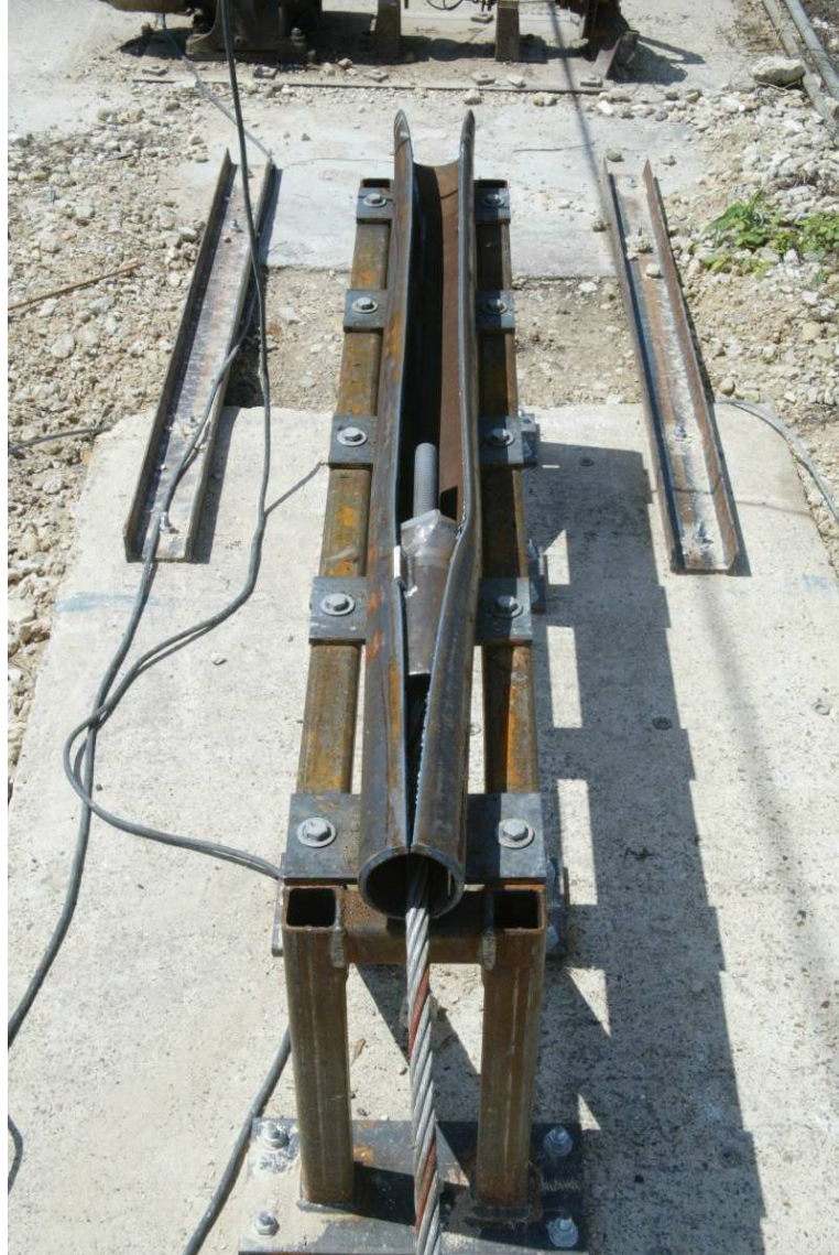
Figure 27. Mandrel Position in Pipe
