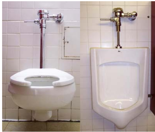
Figure 5: Low-Consumption Manual Toilet and Urinal (Hwan, 2003)
