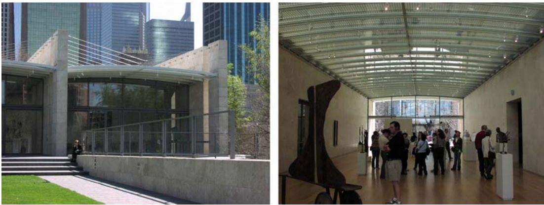
Figure A 6 Exterior view (left) and interior view (right)
