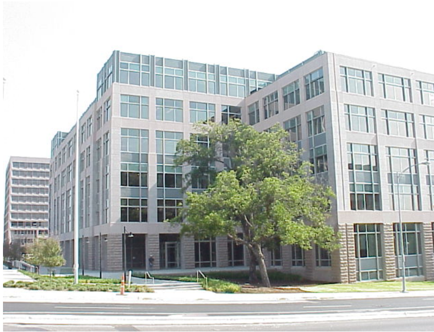
Figure 24: . Entrance View of the Robert E. Johnson building From the Southwest Corner.
