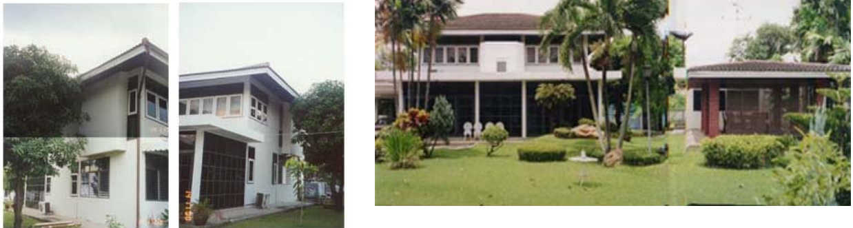
Figure 55: Case study house in Thailand.
