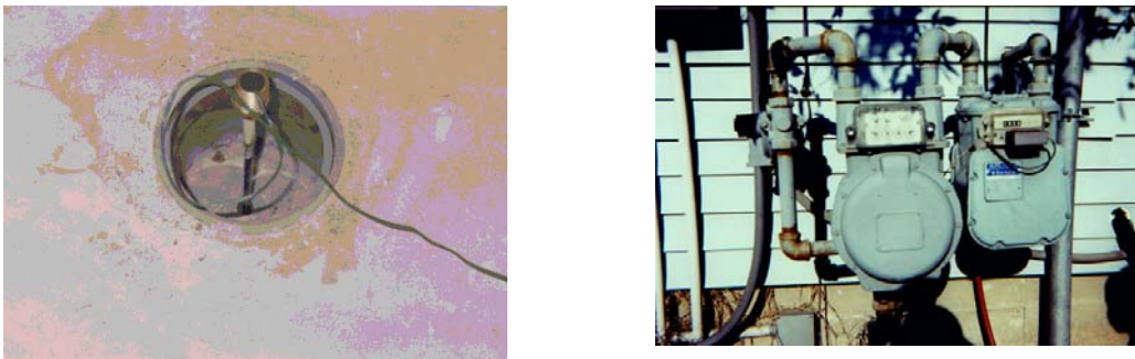
Figure 61: Data logger and natural gas metering.
