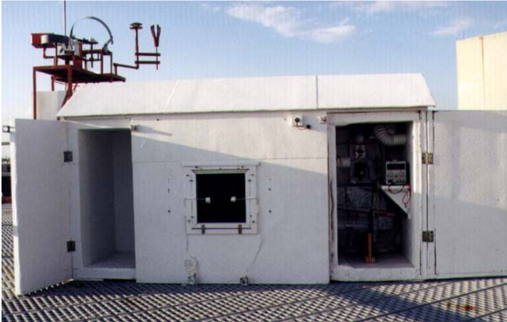
Figure 38: Test facility for shaded fenestration.
