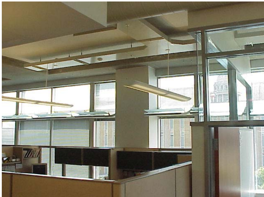
Figure 25: View of windows on south side of building showing light shelf, lighting, and office furniture.
