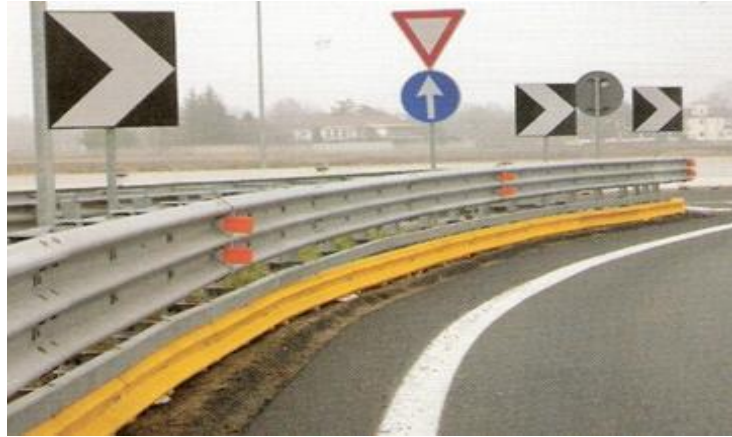
Figure 2.15 Conforming Barrier – Spanish Guardrail (Reprinted from FHWA, 2012).
