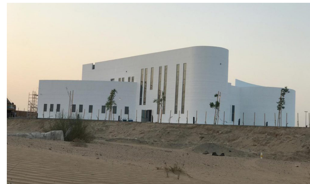
Dubai Municipality Building Elevation
