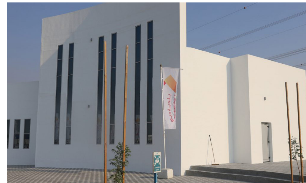
Dubai Municipality Building Elevation
