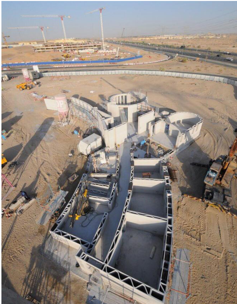
Dubai Municipality Building Construction
