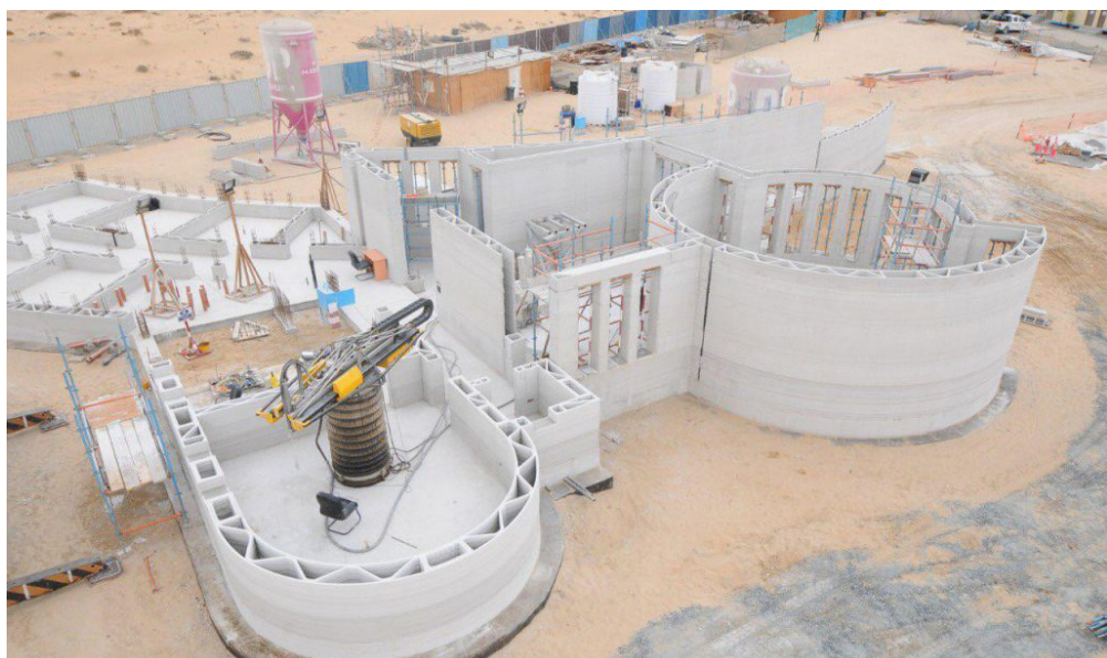
Dubai Municipality Building Construction
