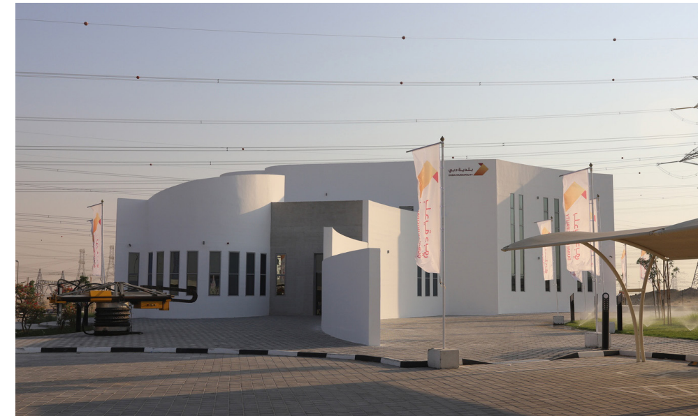
Dubai Municipality Building Elevation
