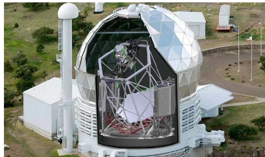
Hobey-Eberly Telescope Cut Showing Telescope
