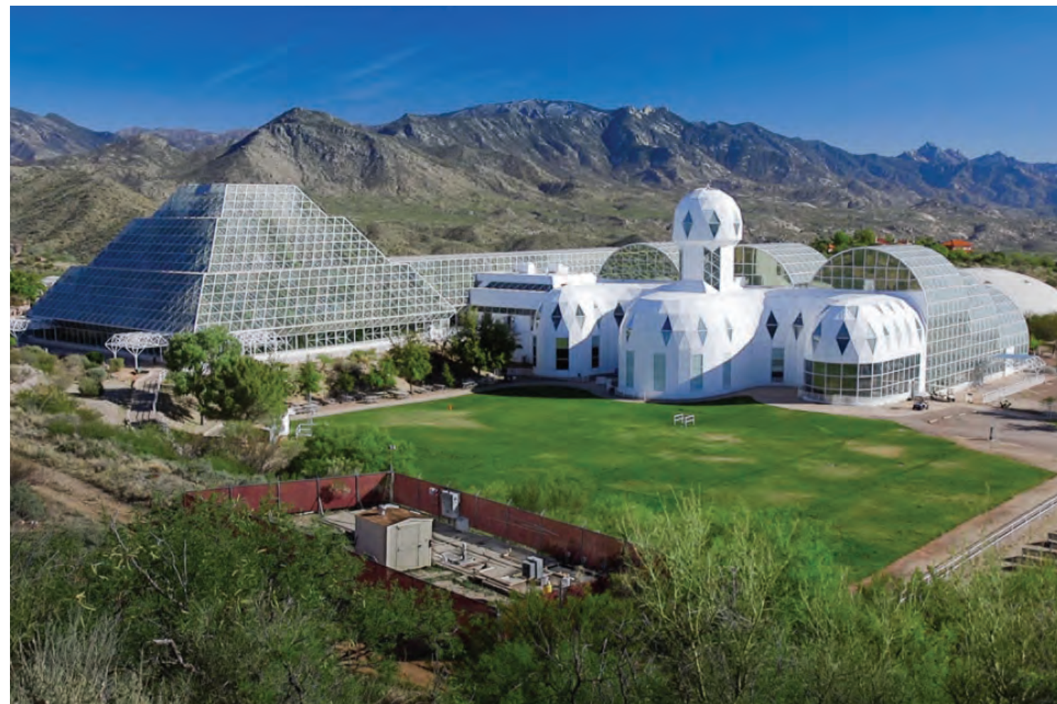
Figure 7 - View of the Biosphere 2 facility
