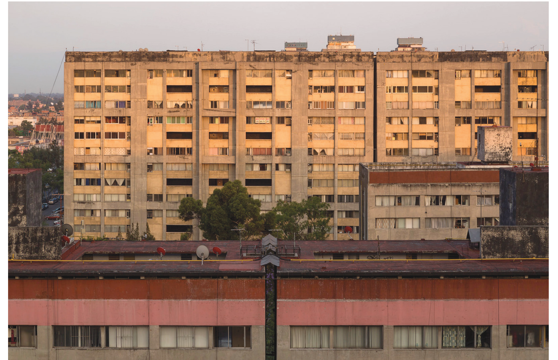
TLATELOLCO HOUSING COMPLEX // MEXICO CITY, MEXICO.
