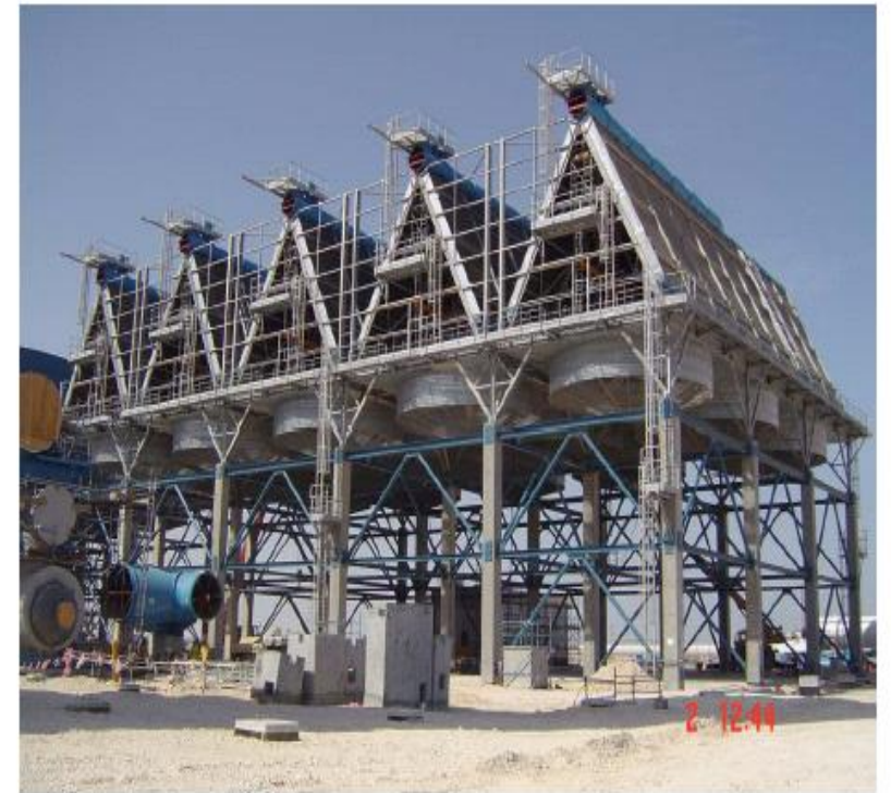
ACC under construction
