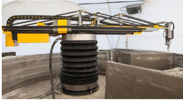
Figure 8. Robotic arm with a concrete extruder developed by Apis Cor [6]
