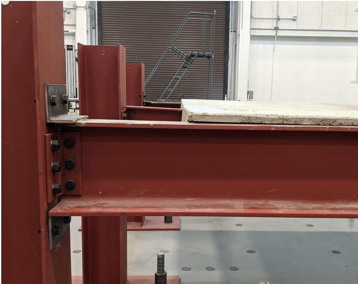
Figure 5.48: Center beam deformation and steel-concrete separation (Photo by Matthew Yarnold)
