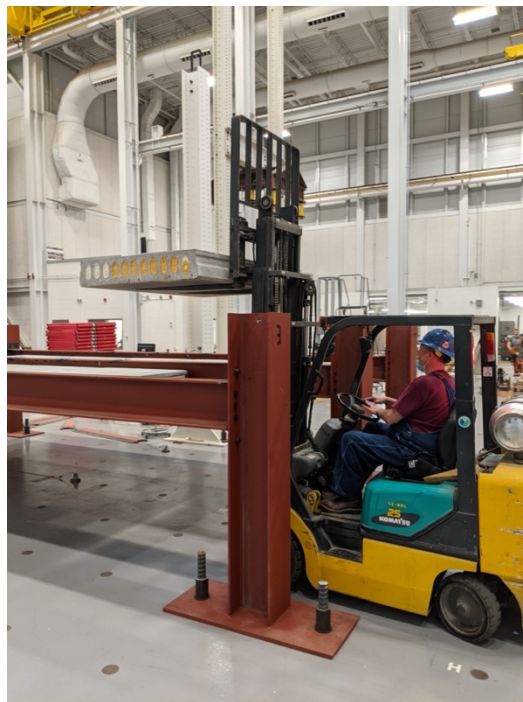
Figure 4.18: Forklift lifting precast panel (Photo by Matthew Yarnold)
