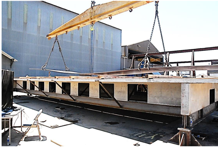
Figure 3.11: Prefabricated composite floor-building system [18] 1
