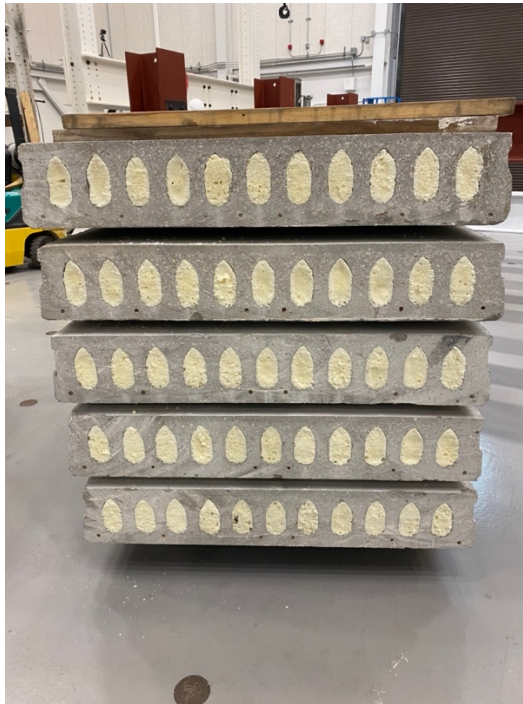
Figure 4.17: Filled hollow-core panels (Photo by Sheyenne Davis)
