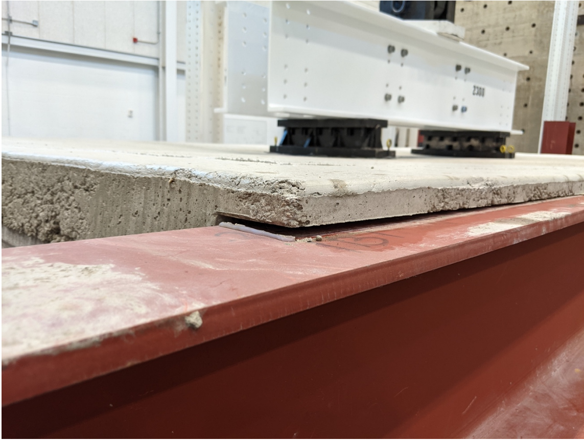
Figure 5.49: Concrete deck separation from steel beam (Photo by Matthew Yarnold)
