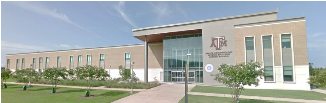
Figure VI-7 Exterior view of the case study building (Retrieved from Google Images)
