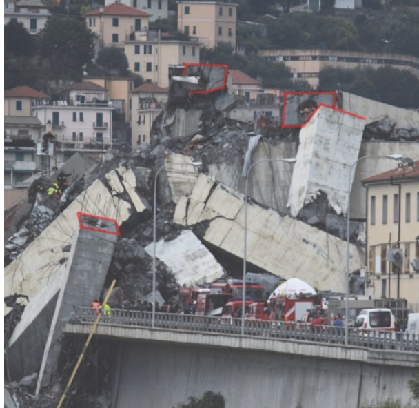
Figure 2.3: Collapse of the Polcevera Viaduct, reprinted from (Bazzucchi et al., 2018) with permission.
