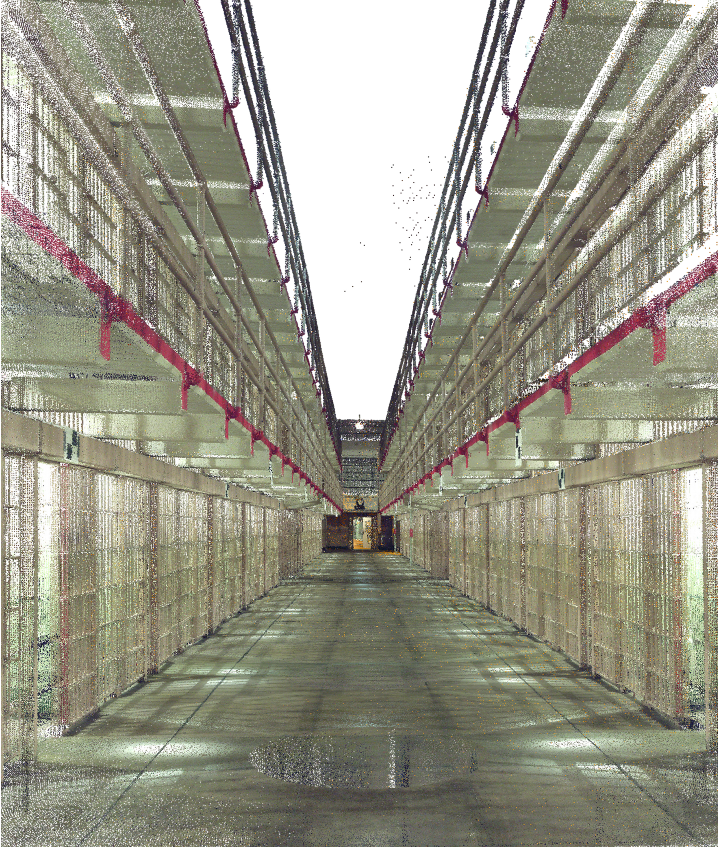
Figure 16: C Block [From block center looking North]
