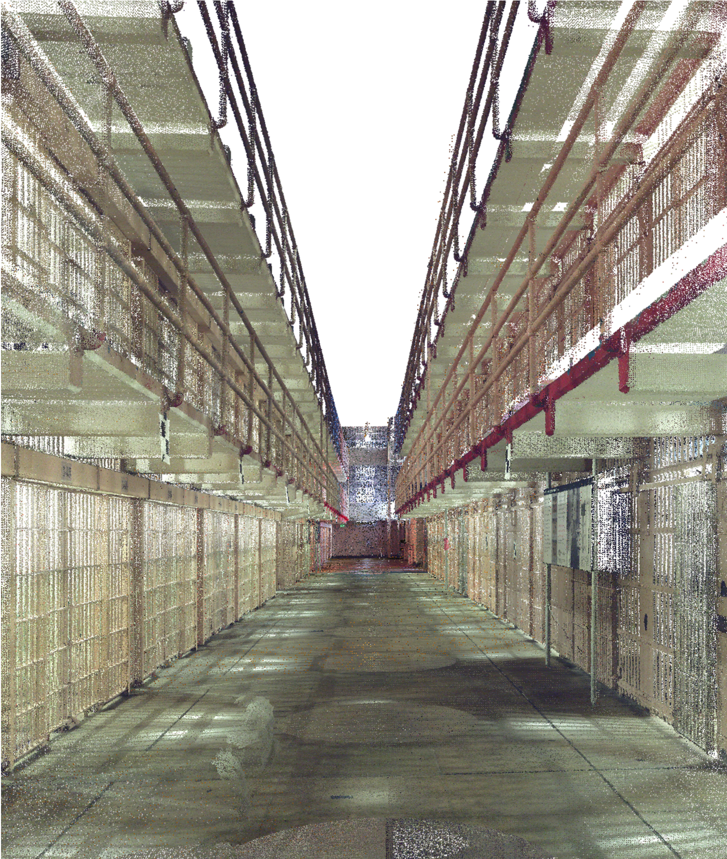
Figure 15: B Block [From block center looking North]
