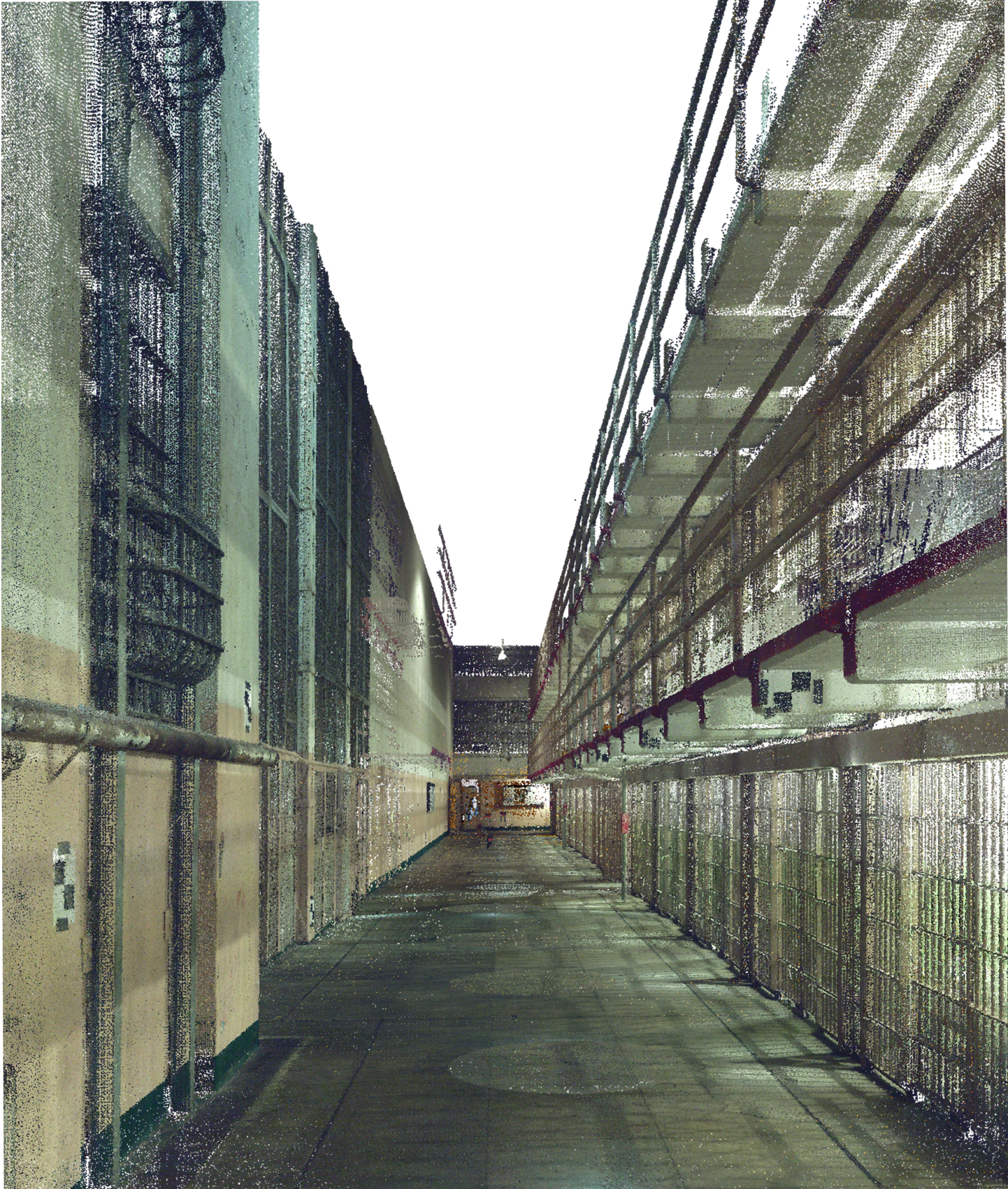
Figure 17: D Block [From South end looking North]
