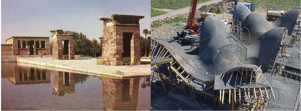
Figure 9. (left) Temple of Debod in the late 90s [img src: Arnold 1999], (right) Bosjes Chapel formwork and reinforcement during application of shotcrete [img src: PERI Group].
