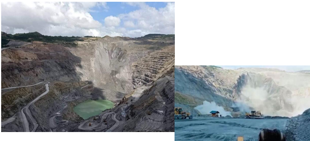
Figure 1.3 Slope failure occurred at Carmen Copper mine (Philippines) on 21 December 2020 (Image tweeted by News5)
