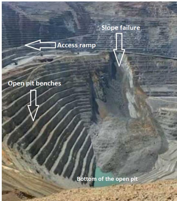
Figure 2.4 Slope failure in the open pit mine (photo by FOX 13)
