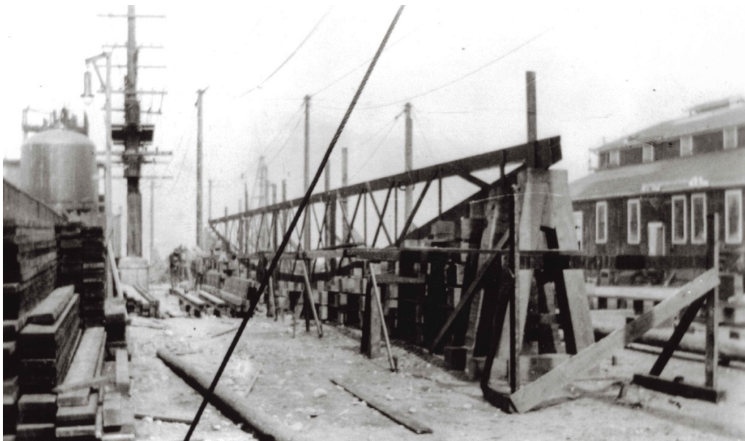
Figure 51. Barnet building ways.
