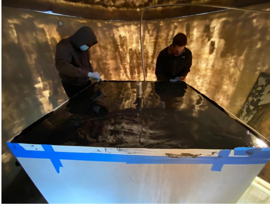
Figure 20. Applied FlexSeal layer
