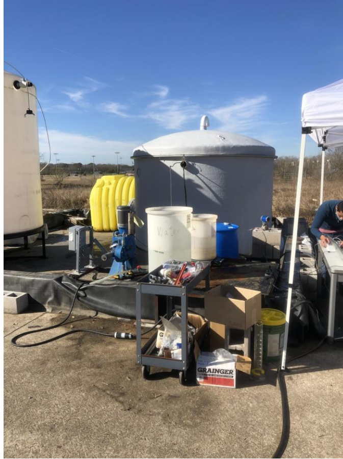
Figure 23. Experimental setup during construction
