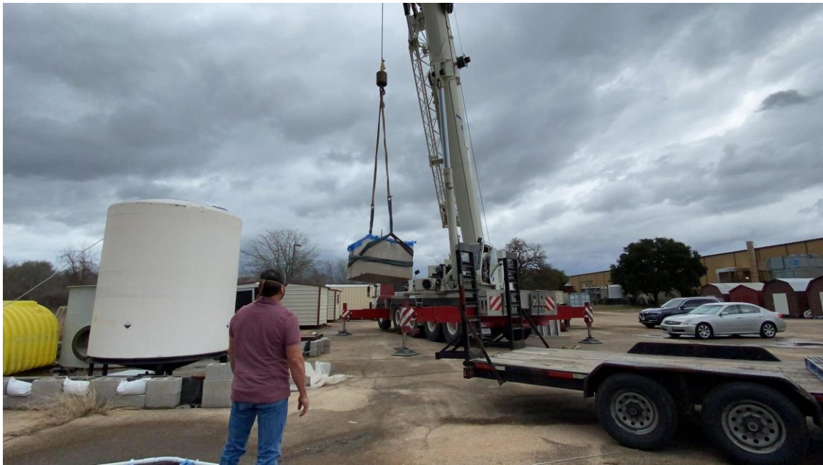
Figure 36. Block removed from tank after acidizing
