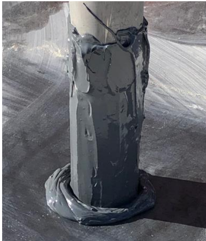
Figure 11. Pipe coated with epoxy layer
