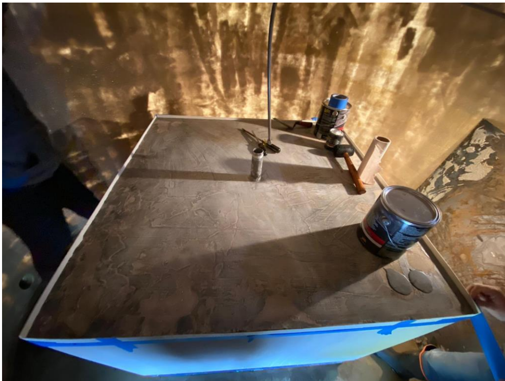
Figure 19. Preparation for FlexSeal epoxy
