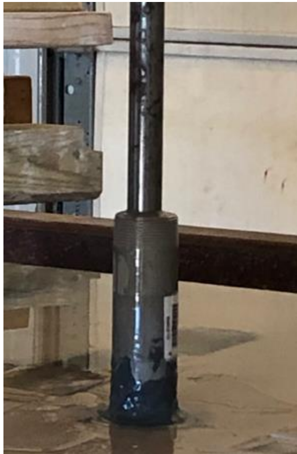
Figure 12. Coring machine in use for open hole
