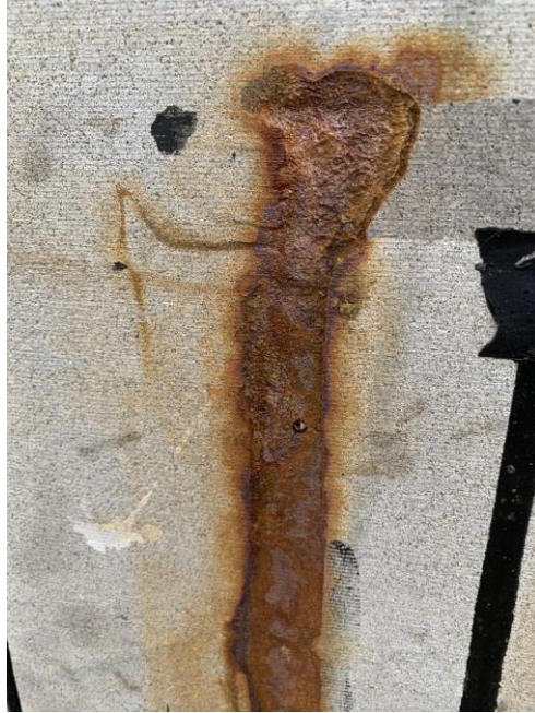
Figure 37. Acid stain on block
