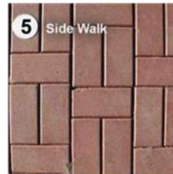
5 Side Walk Porous pavers
