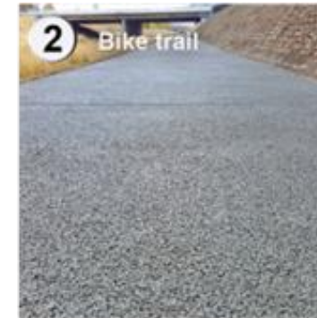
2 Bike trail Pervious Concrete
