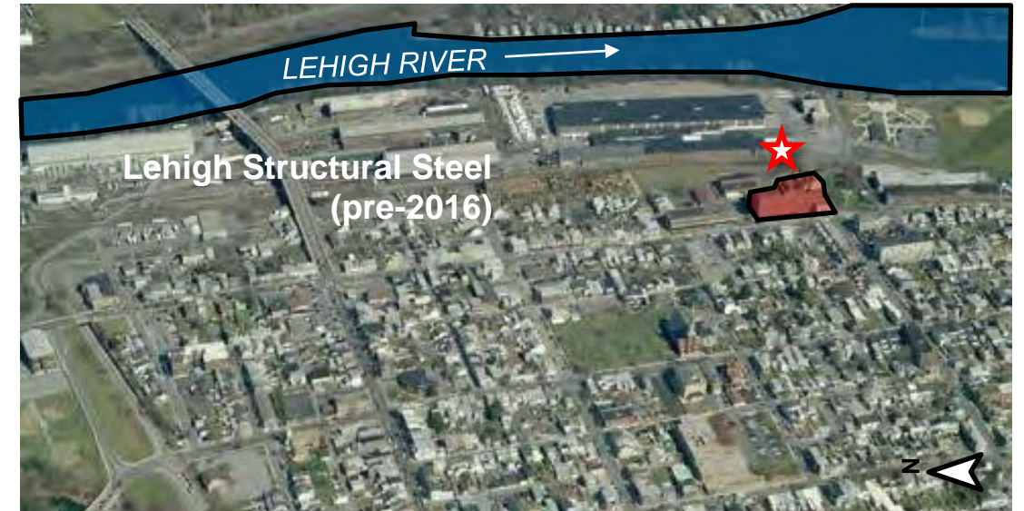
Closed industrial buildings along riverfront, the "Industrial Curtain"
