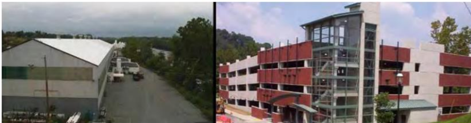
Existing Lehigh Structural Steel site and vision for future parking structures
