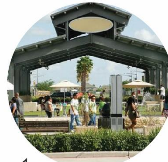
1 metal roof open-air pavilion
