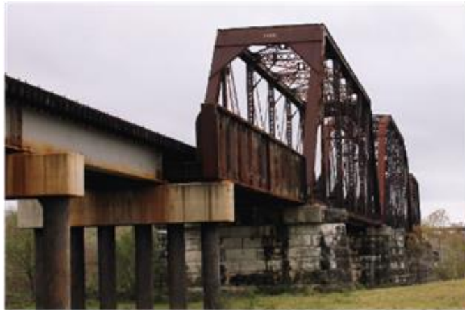
Texas and New Orleans Railroad Bridge
