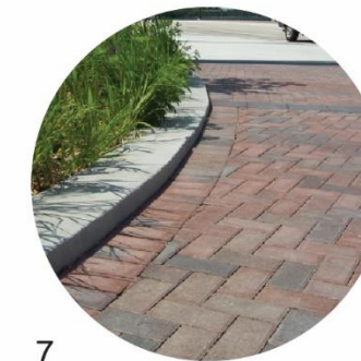
7 interlocking permeable pavers in herringbone pattern
