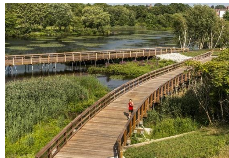
Wetland with Elevated Walkway
