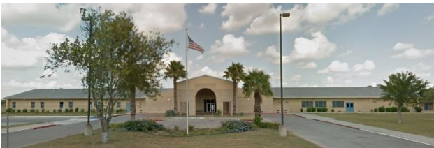
Figure: LC Smith Elementary School (a) Source: Google Street View, 2019
