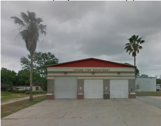
Lyford Fire Department Source: Google Street View 2019
