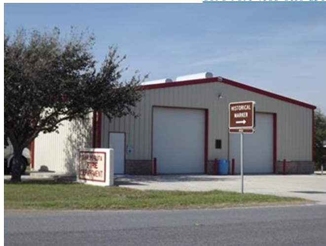
San Perlita Fire Department Source: http://www.waymarking.com/waymarks/WMJXBG_San_Perlita_Fire_Department
