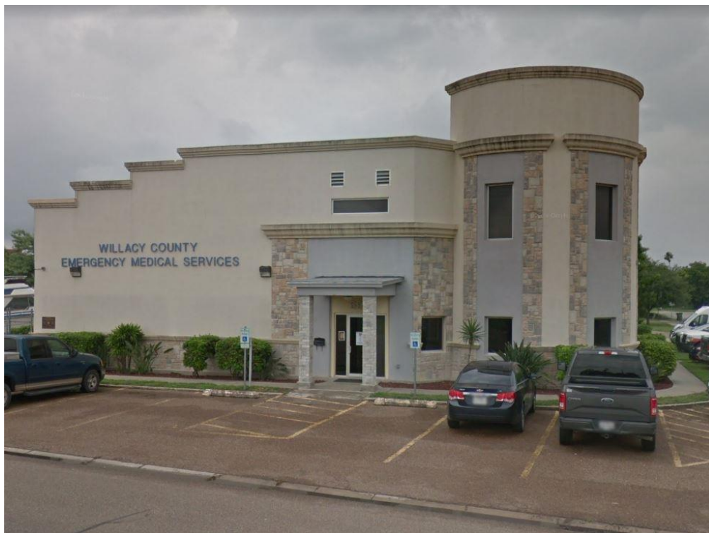
Figure: Willacy County Emergency Medical Services Source: Google Street View, 2019
