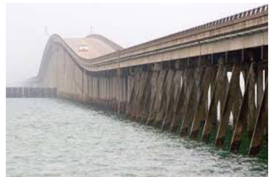
Figure 5.2: Copano Bay Bridge Source: static.tti.tamu.edu
