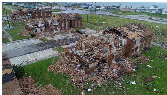
Figure 4.10: Aerial photo of the damage sustained of the Salt Grass Landing Apartments Source: Courtney Sacco and Matt Woolbright 7
