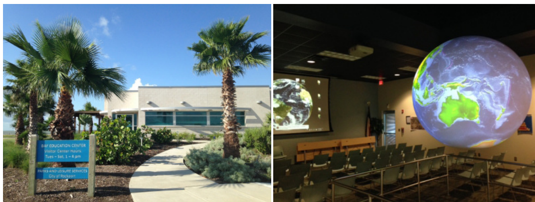
Figure 7.12: Bay Education Center suffered damage in Hurricane Harvey Source: missionaransas.org
