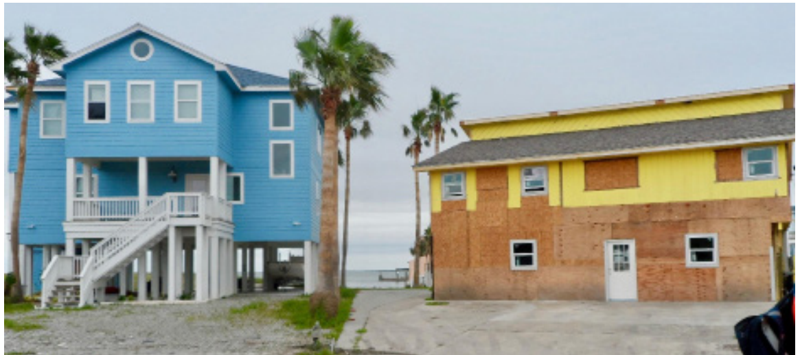
Figure 4.11: Comparison of an elevated home to an unelevated home after Hurricane Harvey Picture Courtesy: Kate de Gennaro
