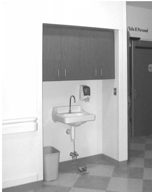
Figure 10: Corridor Sink in the New CCU
