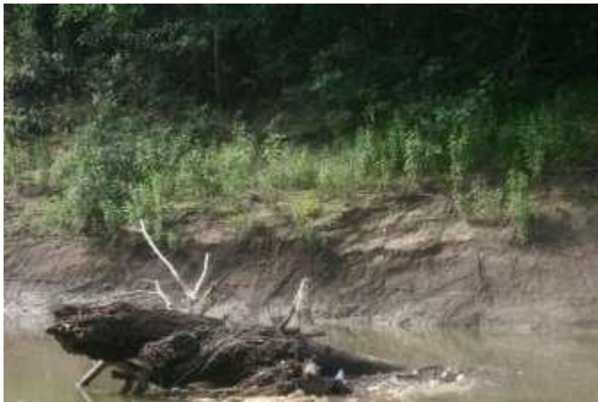
Close-up of bank near Location 4. Bank was extremely clay-rich.
