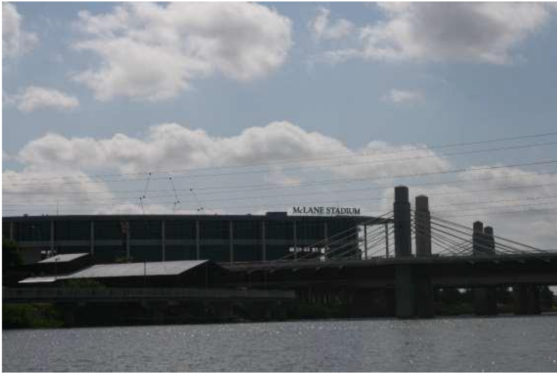
Figure 135: Extensively modified northern bank at BR14.
