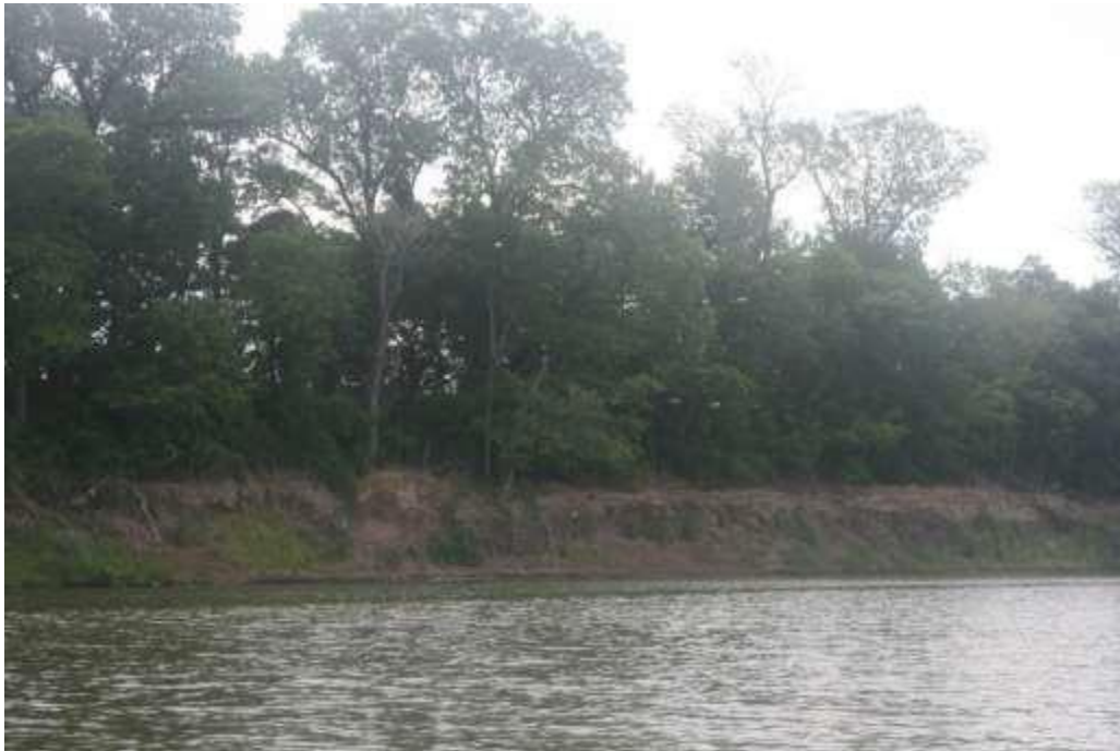
Figure 160: Continuous cuts at BR20
