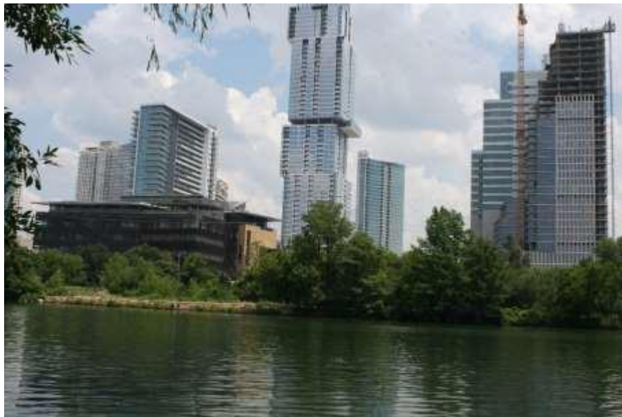
Figure 10: Colorado River channel in Austin, Texas, exhibiting wooden stabilization structures.
