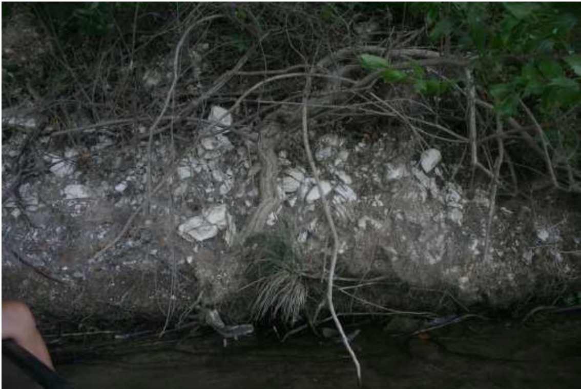
Figure 120: Cutting at BR09
