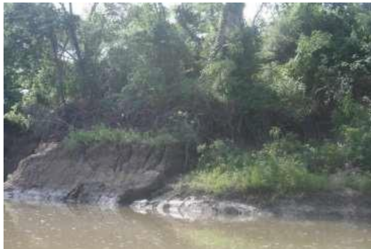
Figure 212: Small slump near Stop 2
