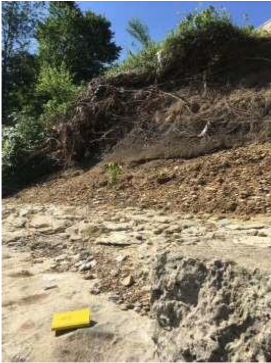
Bank sediment at put-in, Santa Fe Trestle
