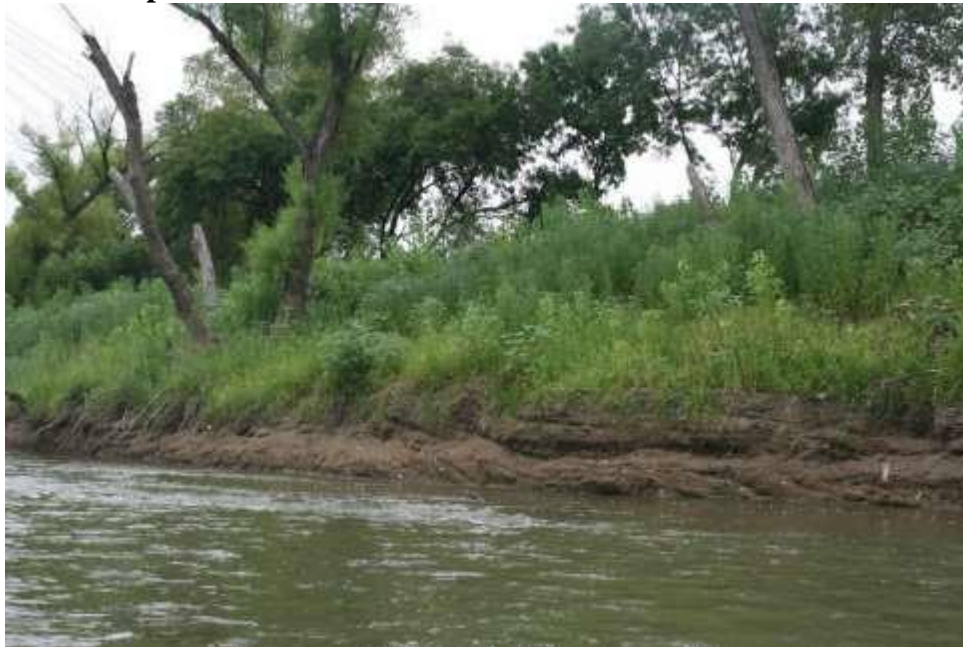
Figure 194: Scalloping layers on southern bank at TR06 TR07
