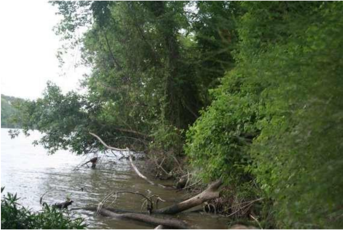
Figure 124: Well-vegetated northern bank at B11, though some trees are leaning.
