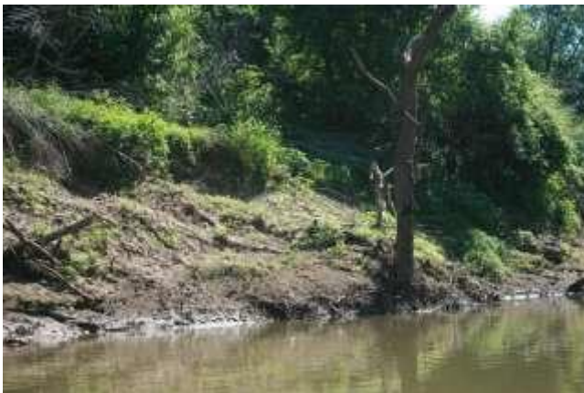
Recent earthflow at Location 4.
