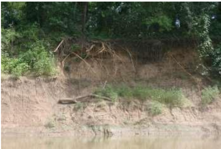
Figure 216: Banks near Location 6
