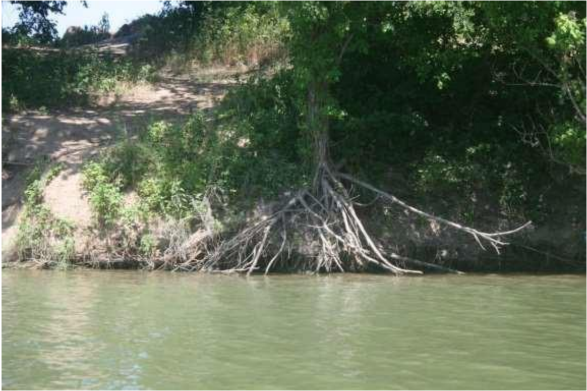
Figure 119: Increased erosion observed near the FM 3051 overpass
