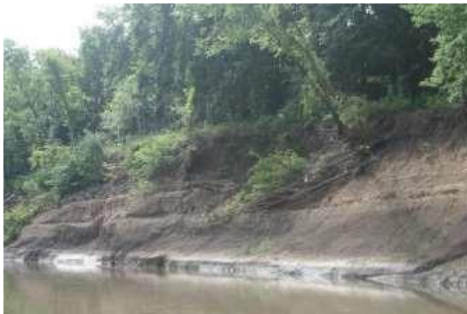
Bank near Location 4; notice leaning vegetation closest to bank, small slump to left of frame
