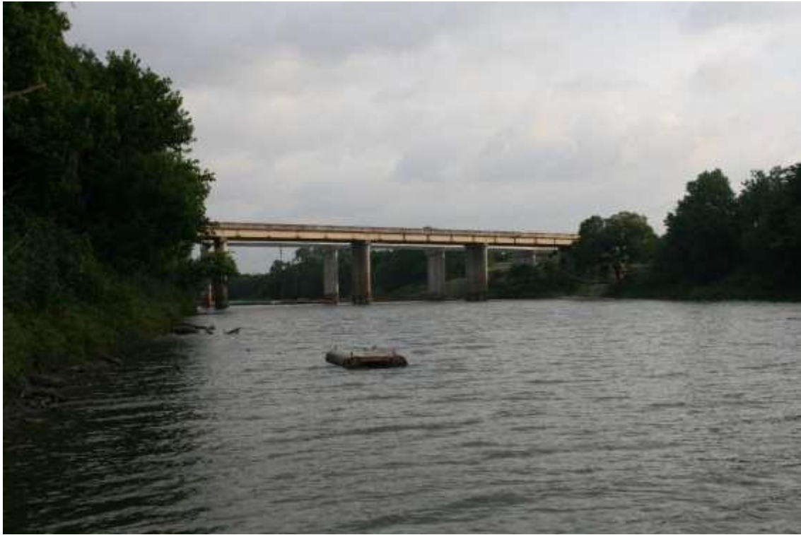
Figure 145: TX-6 overpass, some anthropogenic debris
