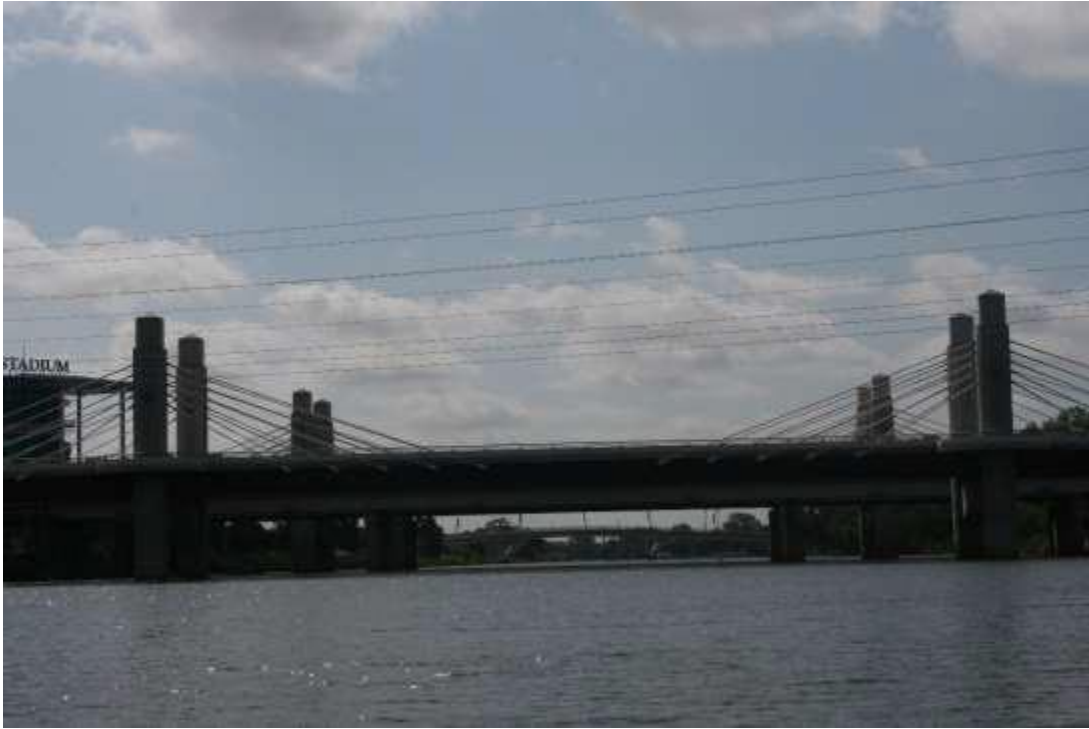
Figure 137: Open channel with no debris, extensive modification.
