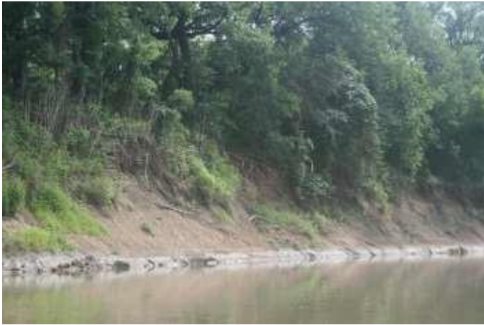
Exposed banks remain prevalent in some stretches near Location 6.
