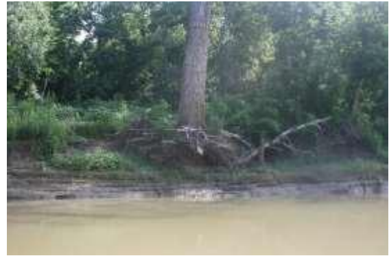
Figure 208: Exposed roots near Stop 2
