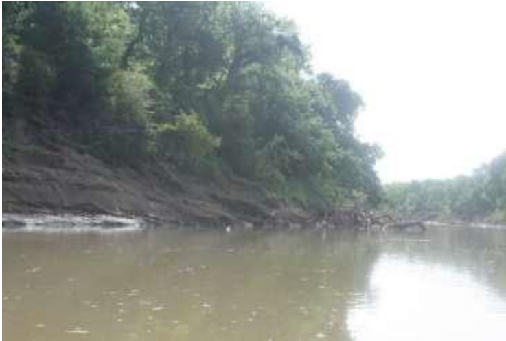
Bank near Location 3; notice exposed bank, slightly angled trees, and debris
