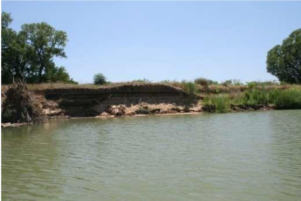
Figure 101: Slump on western bank of BR02
