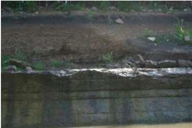
Bedded limestone and bank sediment at Location 4.
