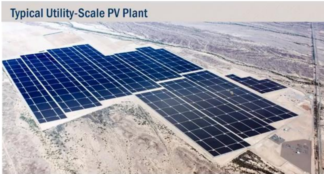
Figure 1-6 Utility scale PV plant in Arizona AGUA CALIENTE 290 MW, AC connection 500 kV in 2010. Reprinted from [10].
