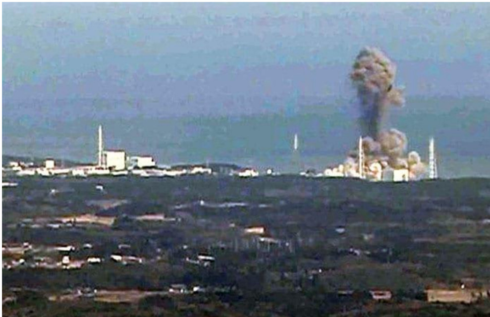
Figure 1. Chemical explosion at Fukushima-Daiichi following hydrogen buildup during a LOCA. Still frame captured from [1].
