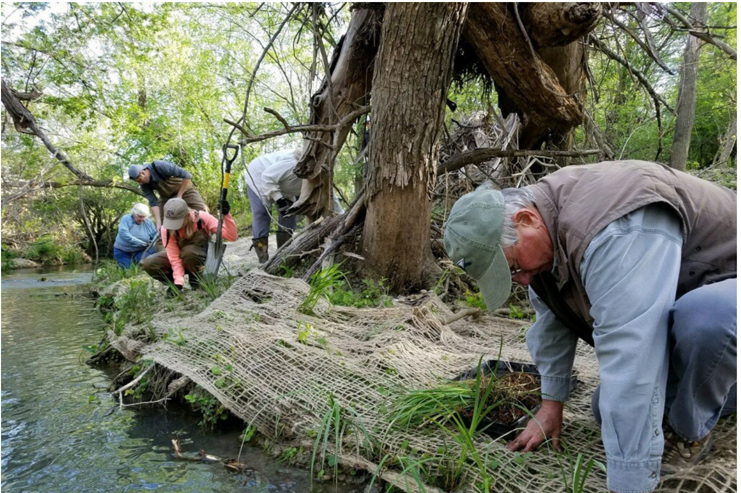
Local volunteers plant obligate plant species near the edge of the water on a portion of the Urban Stream Process and Restoration Program demonstration site at the Irma Lewis Seguin Outdoor Learning Center in the Geronimo Creek watershed in Seguin, Texas. Obligate species thrive in saturated soils and help prevent soil erosion along the bank. Photo by Clare Entwistle, Texas Water Resources Institute.
