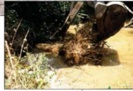
Figure 6.2 Track hoe with hydraulic front-mounted root wad into streambank
