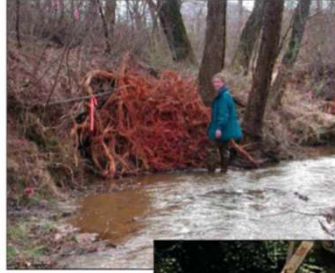
Figure 6.1 Root wad placed on outside of meander bank
