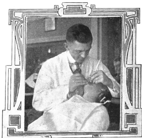
Making Examination to Determine Work Needed.
