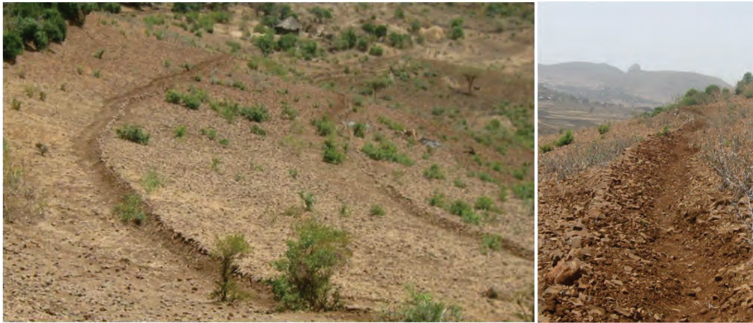
Figure 5. Stone bund treated fields (left image) and the small channel above the stone bund (right image).
