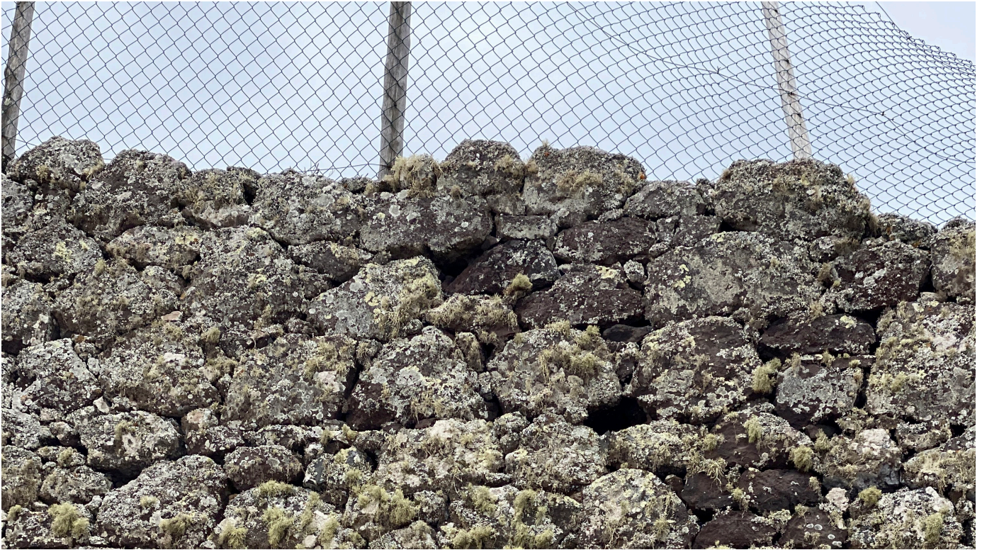
Figure 38: Detail of dry-laid stone wall with bio-growth present (Image: B. Fortenberry).
