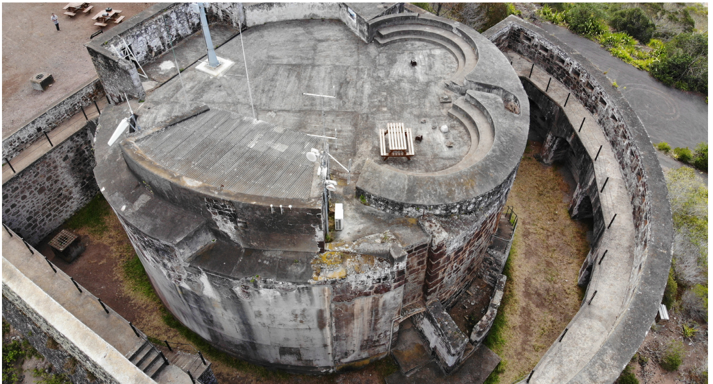
Figure 45: Aerial image of stucco present on the north tower complex (Image: B. Fortenberry).
