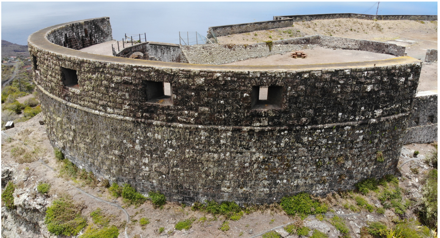
Figure 50: Aerial image of bio-growth on the southern bastion (Image: B. Fortenberry).
