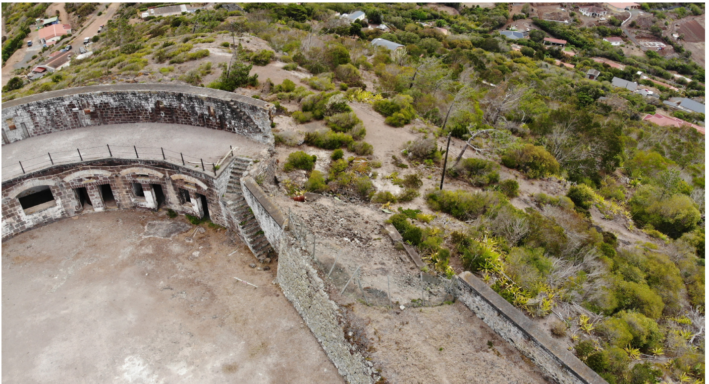
Figure 29: Aerial view of wall collapse in southwest corner looking southwest, interior walls and fence in detail (Image: B. Fortenberry).
