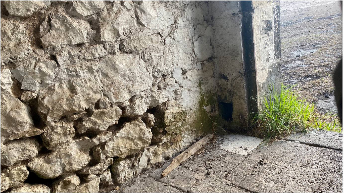
Figure 55: Detail of bio-growth in the barracks in the southern complex (Image: B. Fortenberry).
