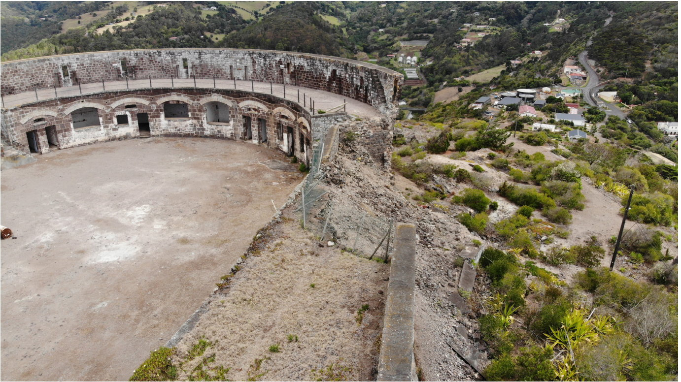
Figure 18: Aerial view of wall collapse from southwest corner of fort looking south (Image: B. Fortenberry).
