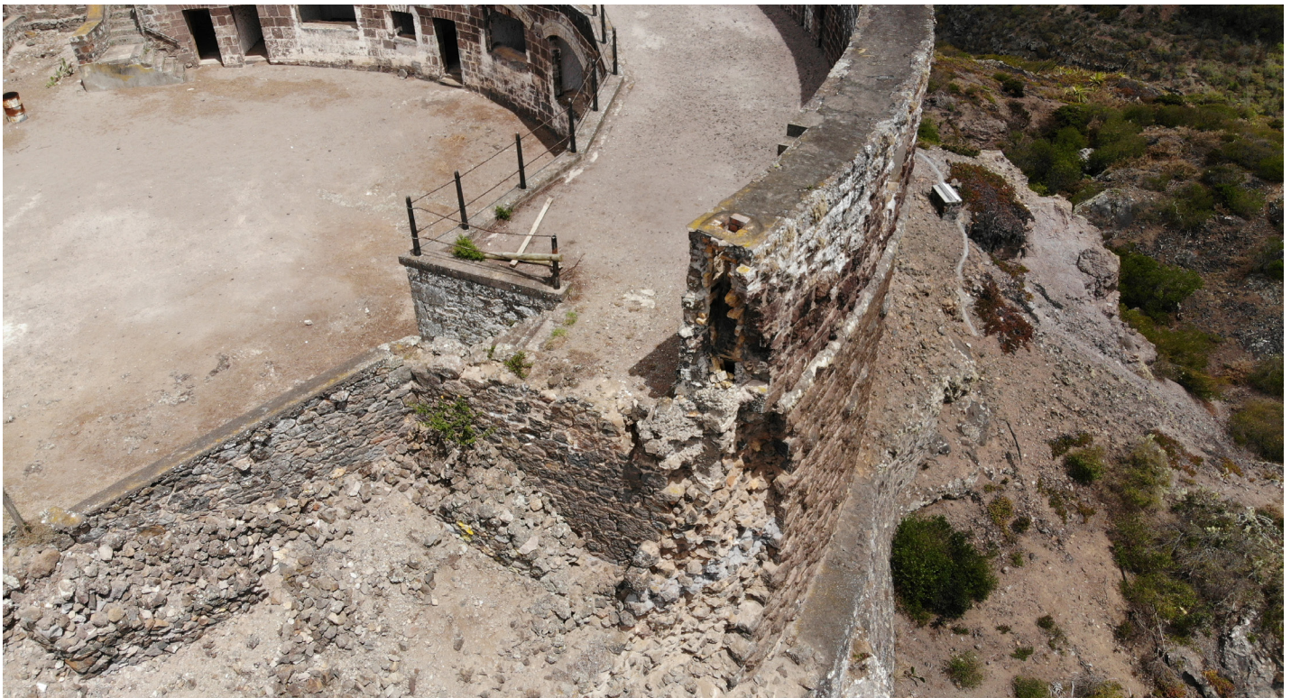
Figure 25: Aerial view of wall collapse from southwest corner with wall section and firing platform in detail (Image: B. Fortenberry).
