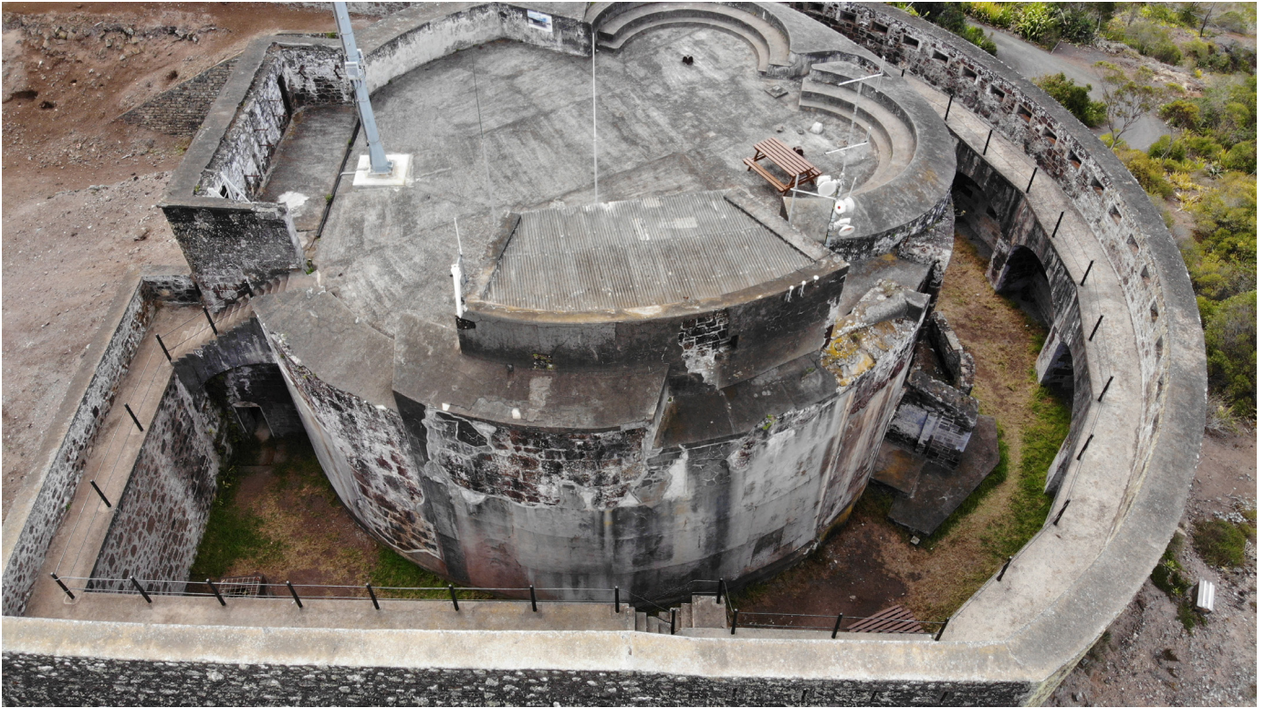
Figure 44: Aerial image of stucco present on the north tower complex (Image: B. Fortenberry).
