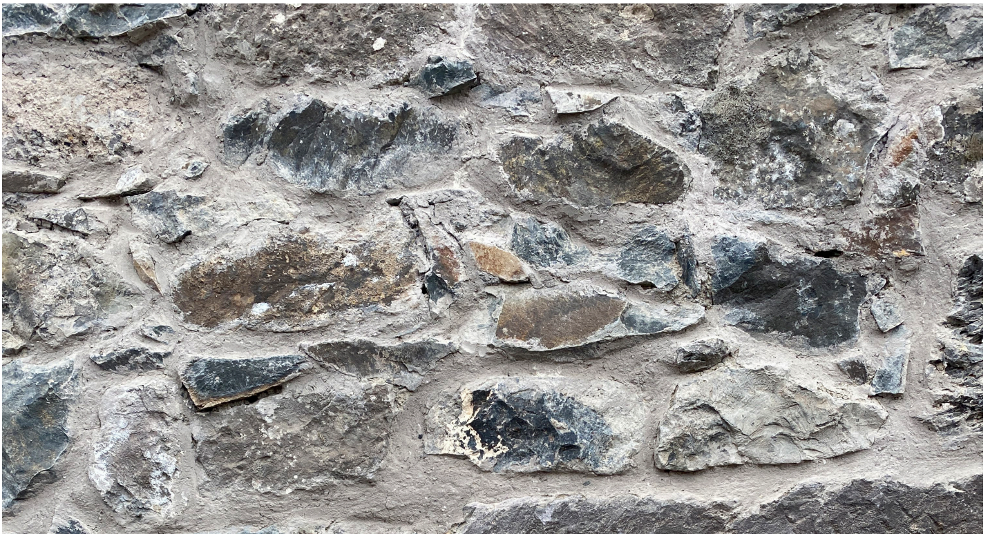
Figure 39: Detail of Portland based mortar without aggregates in detail (Image: B. Fortenberry).
