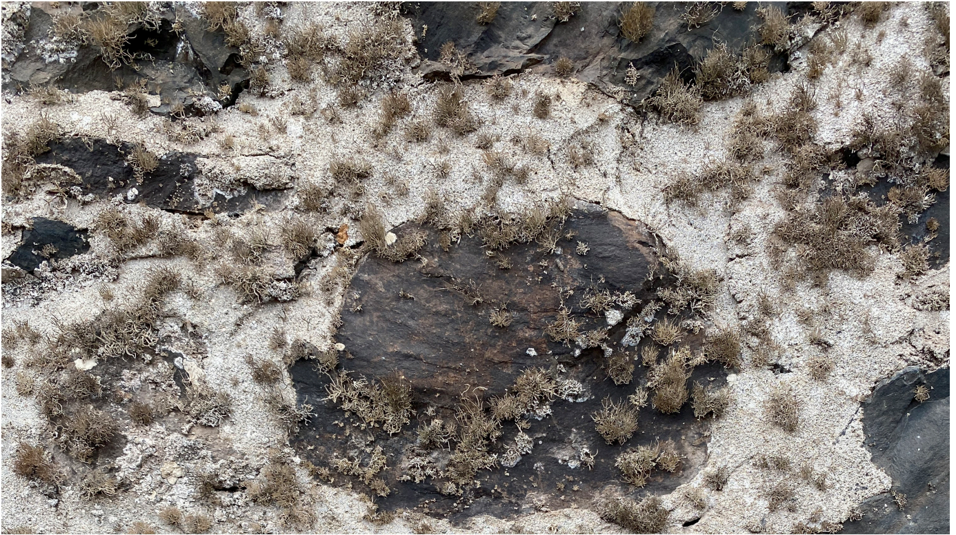
Figure 40: Detail of Portland based mortar without aggregates and bio-growth present in detail (Image: B. Fortenberry).
