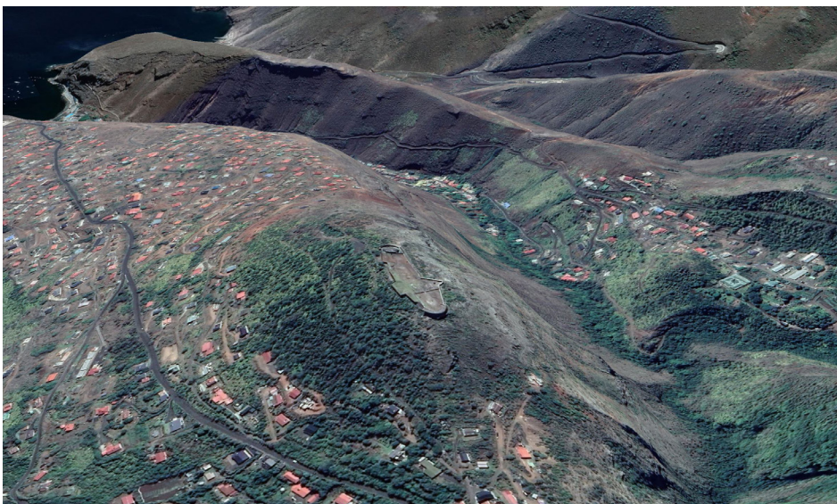
Figure 5: Oblique 3D Google Earth Imagery of High Knoll Fort (Image: Google Earth)
