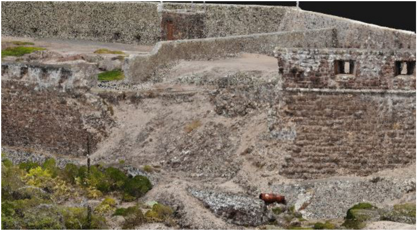
Figure 16: Photogrammetric detail of wall collapse (Model: B. Fortenberry).
