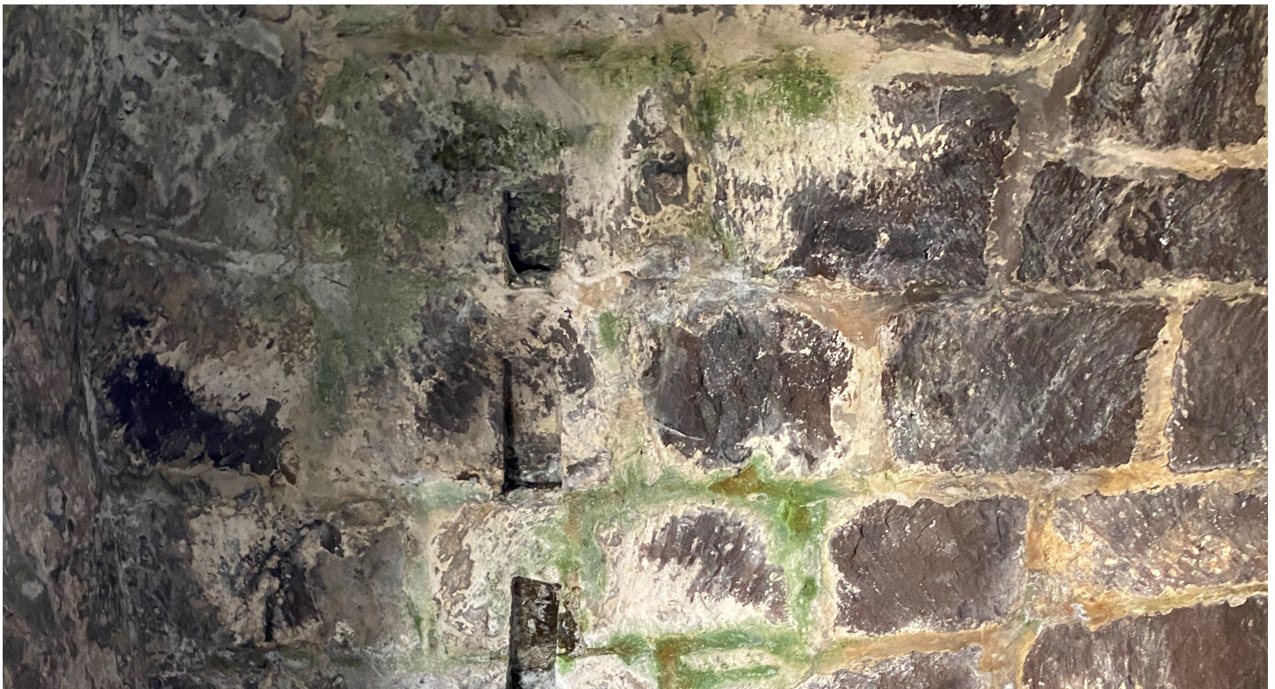
Figure 54: Detail of bio-growth in the magazine in the northern tower (Image: B. Fortenberry).
