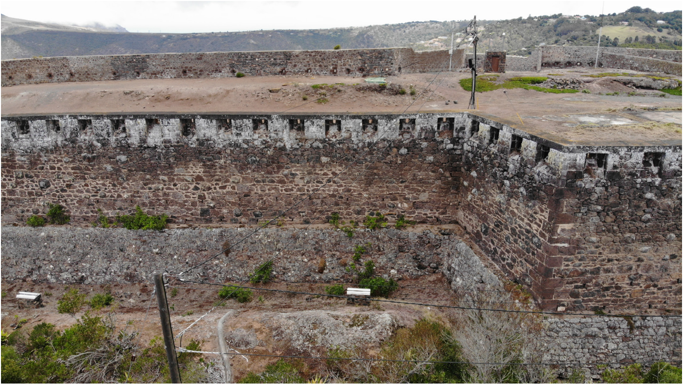
Figure 47: Aerial image of bio-growth on the exterior western wall (Image: B. Fortenberry).
