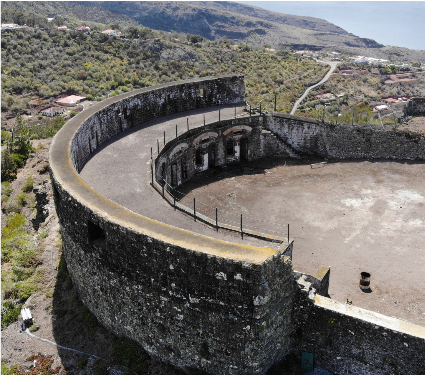
Figure 46: Aerial image of bio-growth on the top surface of the southern firing platform (Image: B. Fortenberry).
