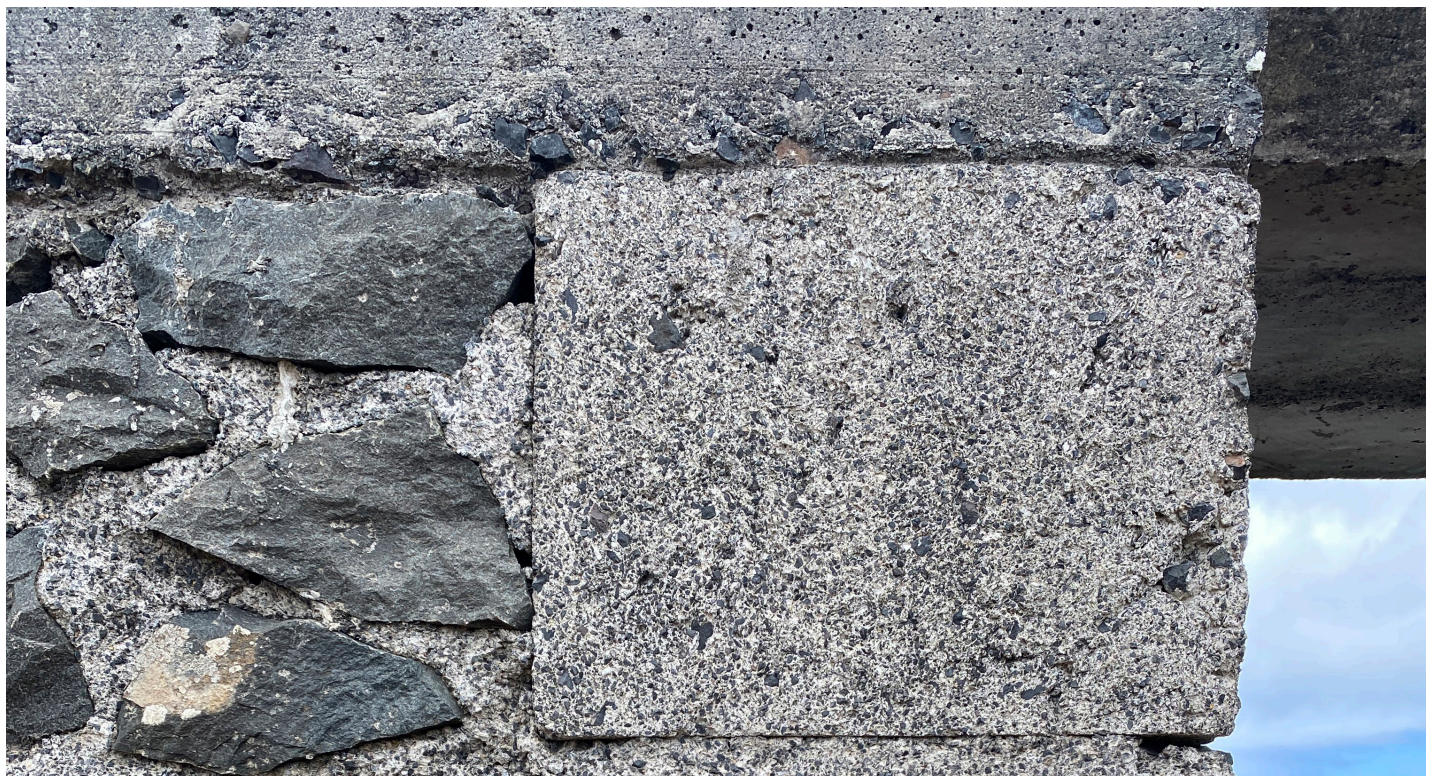
Figure 37: Detail of Portland based mortar in detail (Image: B. Fortenberry).
