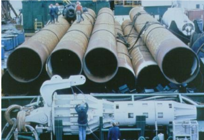
Figure 1.3 Driven Piles, courtesy of Dr. James D. Murff.
