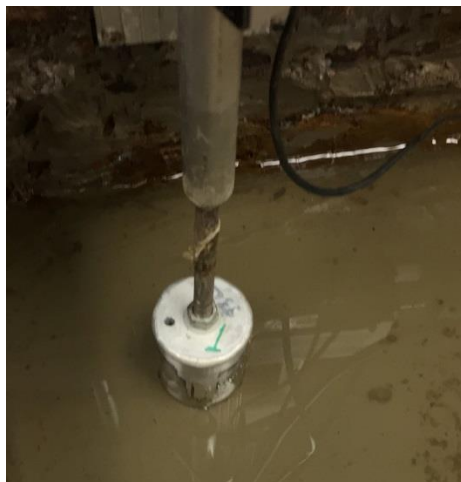
a) Caisson installation (open vent)
