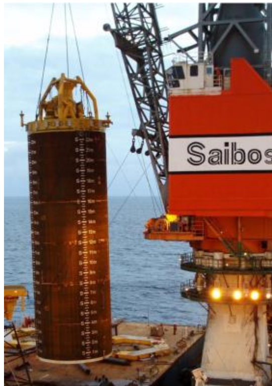
Figure 1.5 Suction caisson (reprinted from Colliat et al. 2011).
