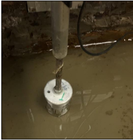
a) Caisson installation (open vent)
