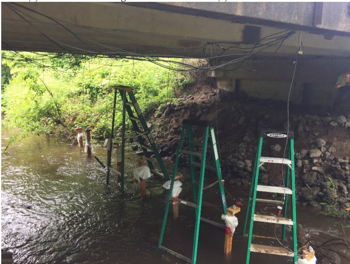
(c) Installed String Potentiometers
