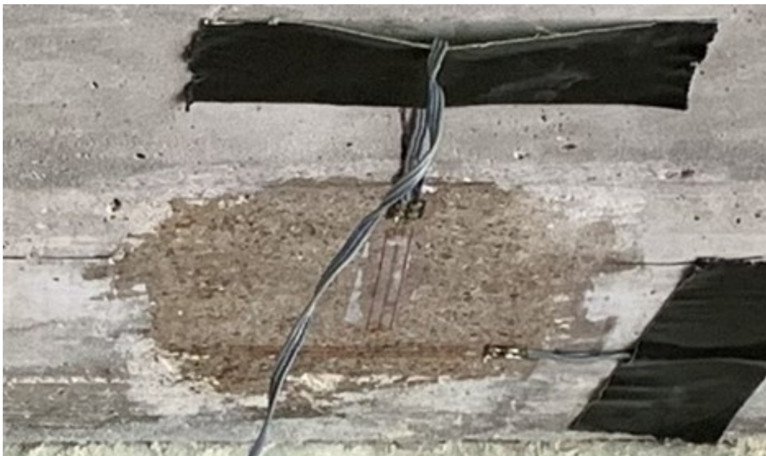
Figure 8.4. Close-Up of Strain Gauge Installation
