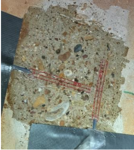
(a) Installed Strain Gauges
