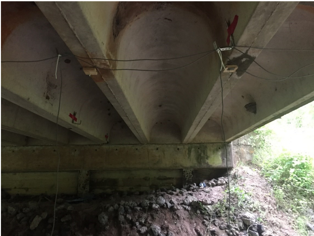
(b) Underside view
