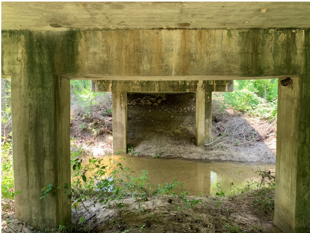
(b) Underside View
