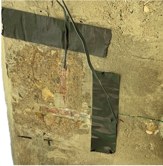
(a) Installed Strain Gauges
