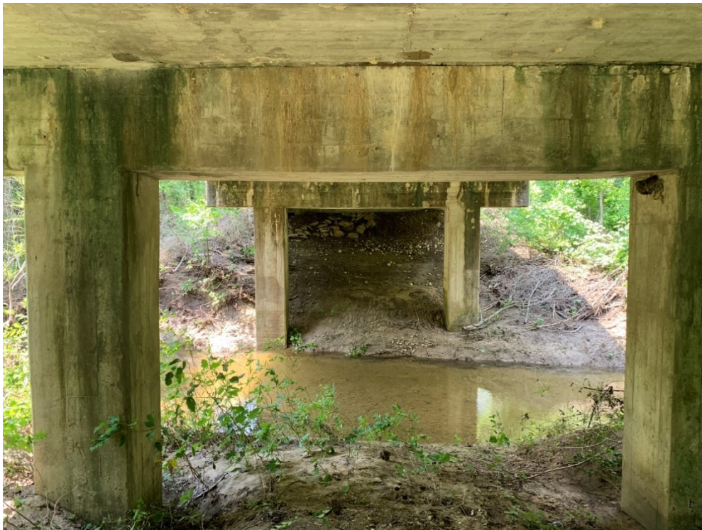
(b) Underside View
