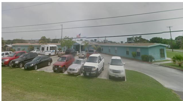
Figure 41. Rockport Coastal Care Center Source: Google Street View, 2017
