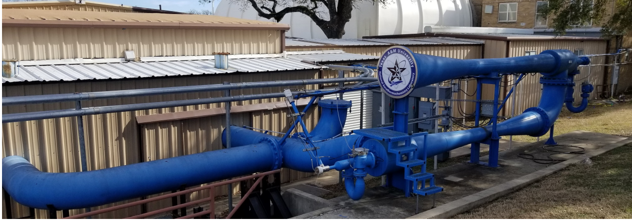
Figure 3.2: Photograph of NAL two-stage ejector system.
