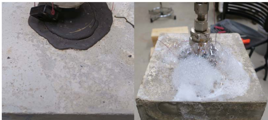
Figure 2.14 Comparison of the localized permeation crack and massive bubble generation from bubble leakage test (Specimen #7).
