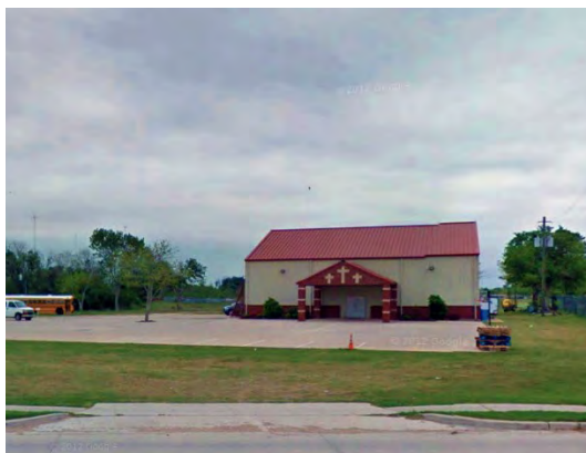
Bethel Church on Fifth Street, across from Fifth Street Community Center
