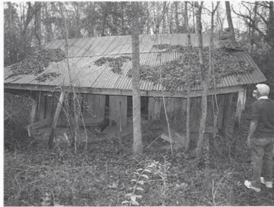
Figure 9. Family rehabilitation of homestead outbuilding, Noah's Ark, 2016. Photograph courtesy Harold Odom.
