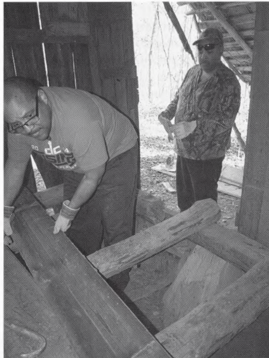
Figure 10. Family rehabilitation of homestead outbuilding, Noah's Ark, 2016. Photograph courtesy Harold Odom.
