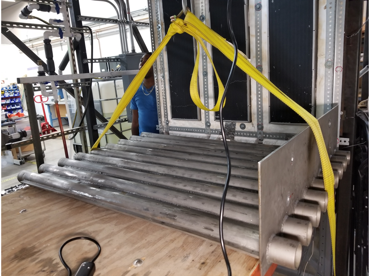
Figure 7.7: Removed cooling panel from WRCCS facility.
