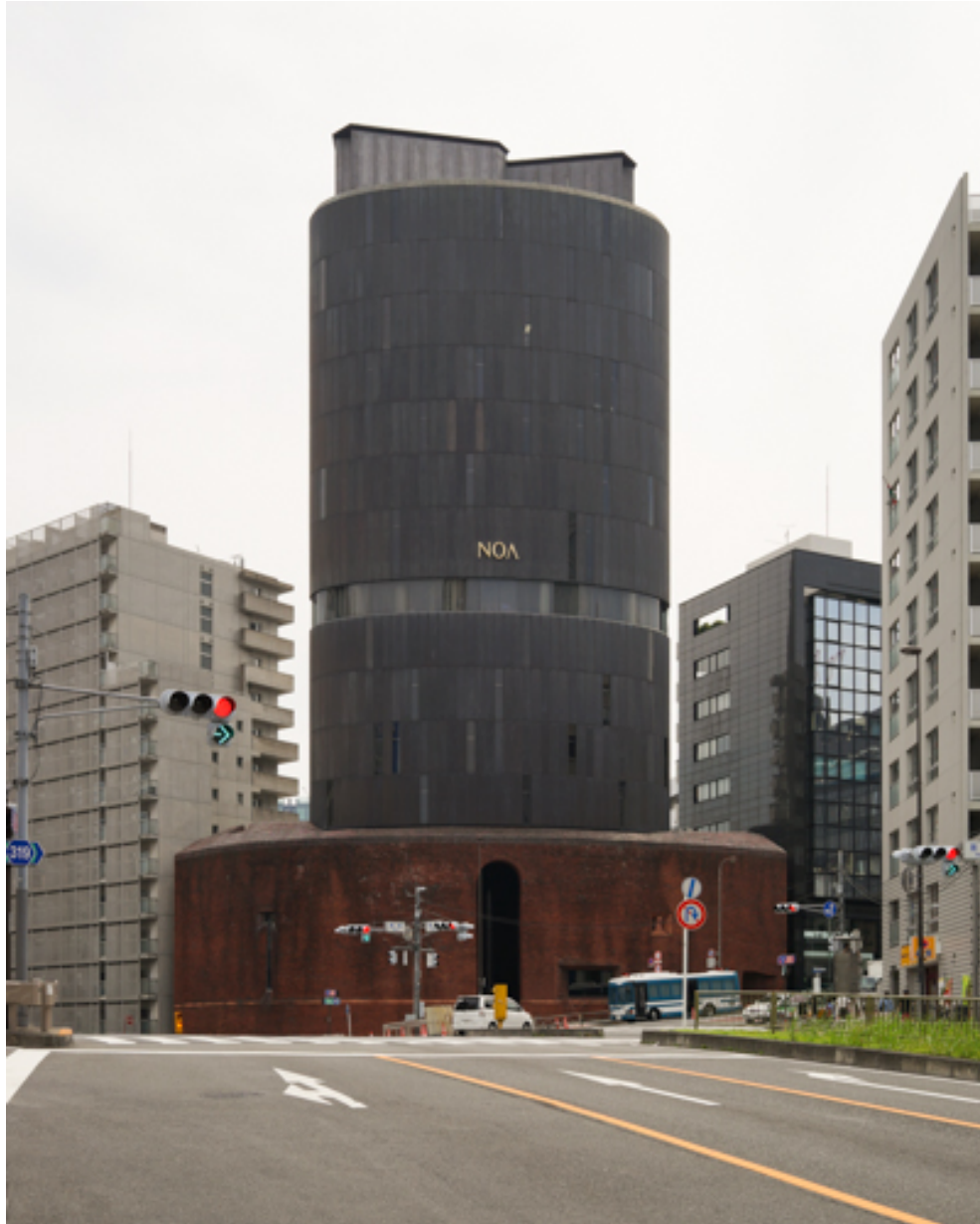
Figure 29: NOA building, elevation (photo by the author)
