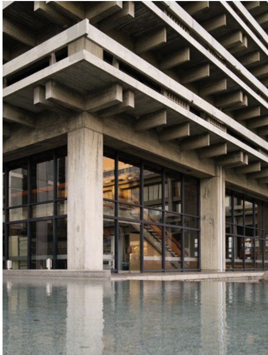
Figure 42: The Kagawa Prefectural Office (photo by the author)
