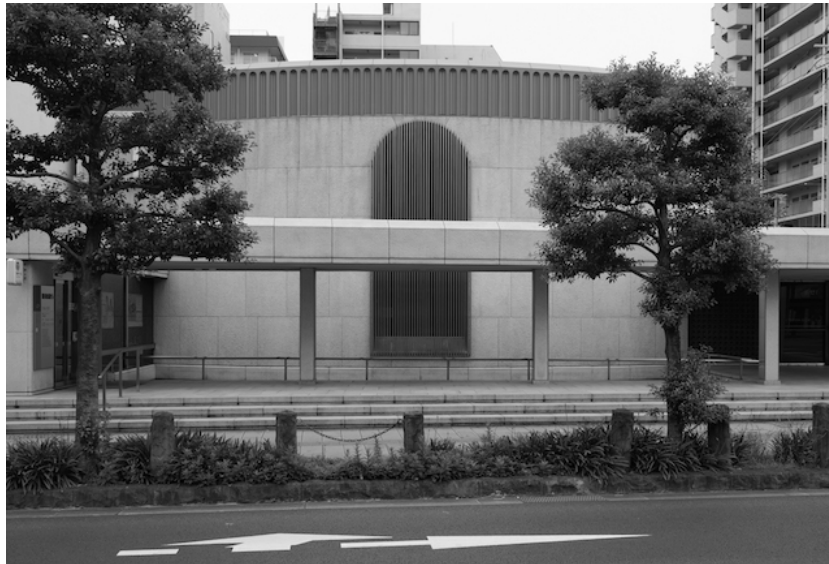
Figure 26: The Ōhato brach of the Shinwa Bank, elevation (photo by the author)
