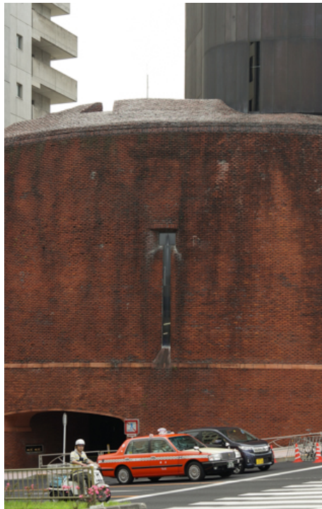
Figure 55: NOA building, facade detail (photos by the author)
