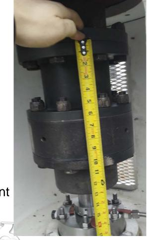
When the suction valve was opened it was noticed that the pump shaft and 4 piece rigid coupling moved about 3/8 inch upward before the pump was started since flow through the pump pushed the components upward.
