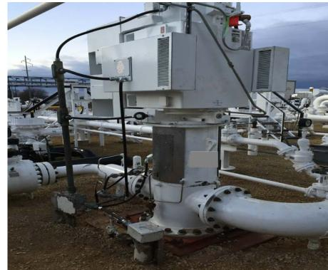
• During a normal pipeline startup the refinery starts up a tank booster pump which feeds the vertical can pump. When pressure is received from the tank pump the vertical can pump is started.
