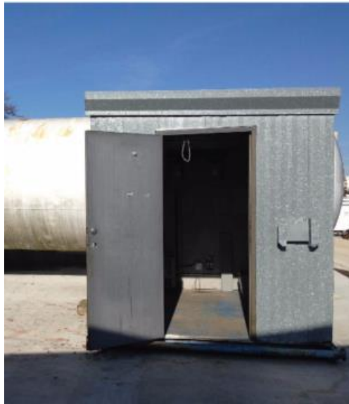
Figure 32: The insulated shed that serves as the facility office.
