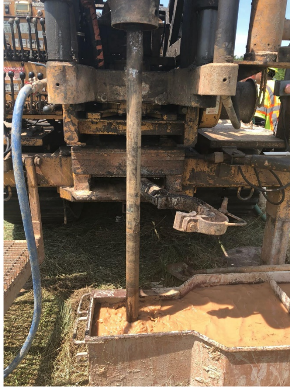
Figure 68. Circulating the drilling fluid in the borehole in order to flush
