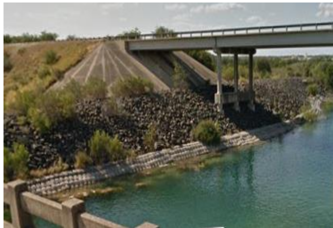
Figure 55- Right abutment repair at US 90 over Nueces River
