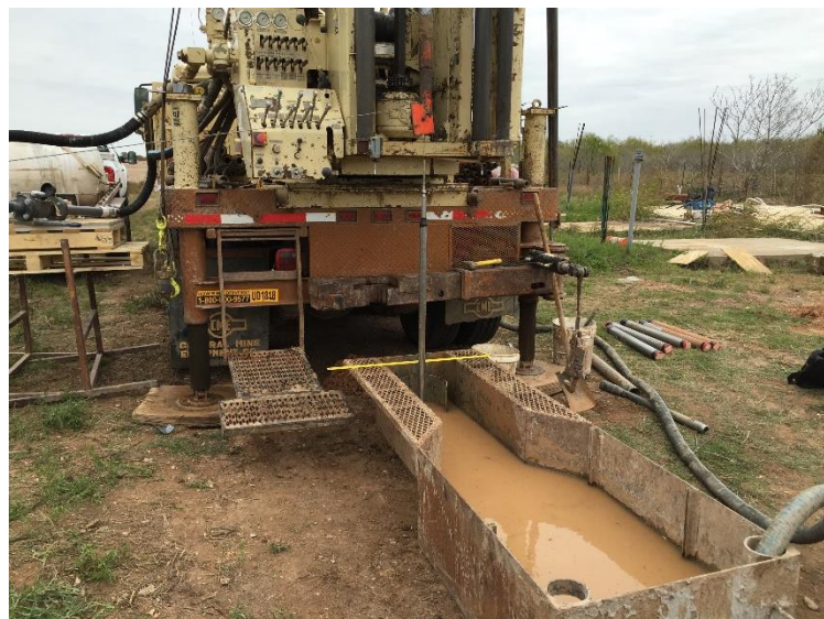
Figure 17- Diameter logging after flow
