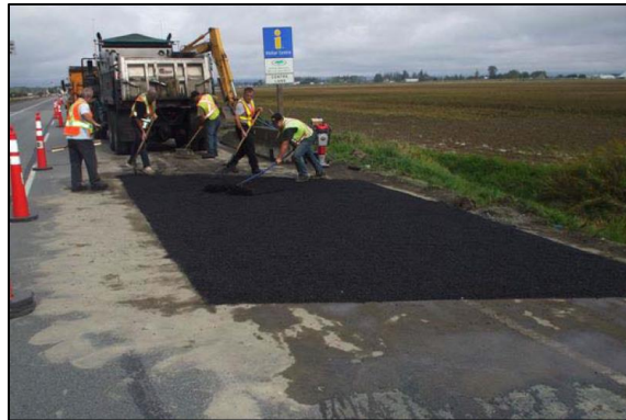
Figure 2. Patching of Road to Repair Pavement Distress. Reprinted from [7].
