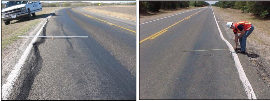
Figure 1. Instance of Deep Rutting and Severe Rutting. Reprinted from [7].
